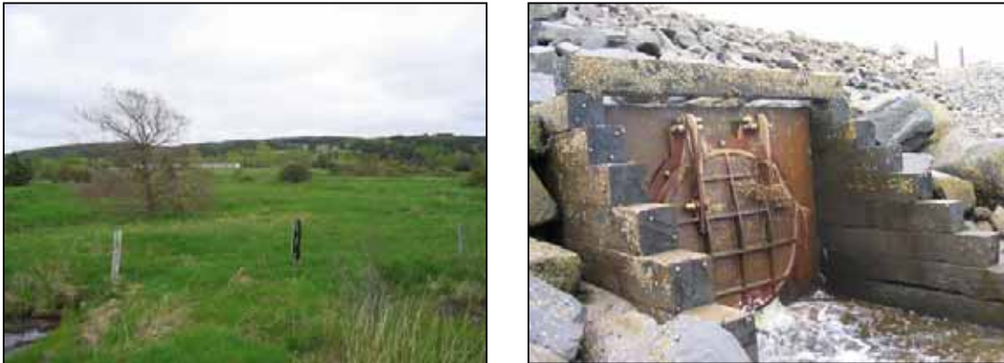
Figure 7: Landward view of restorable area (left) and downstream view of aboiteau (right)
