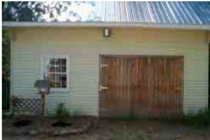
Outside - Air Intake and Rain Shelter
