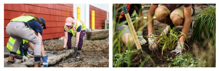
The project involved the removal of over 200 m2 of unused pavement and the installation of native plants to aid in the absorption of stormwater runoff from surrounding impervious services, such as the parking lot and nearby building. Over 300 plants were planted in the rain garden with the help of community volunteers, including youth from local schools.
