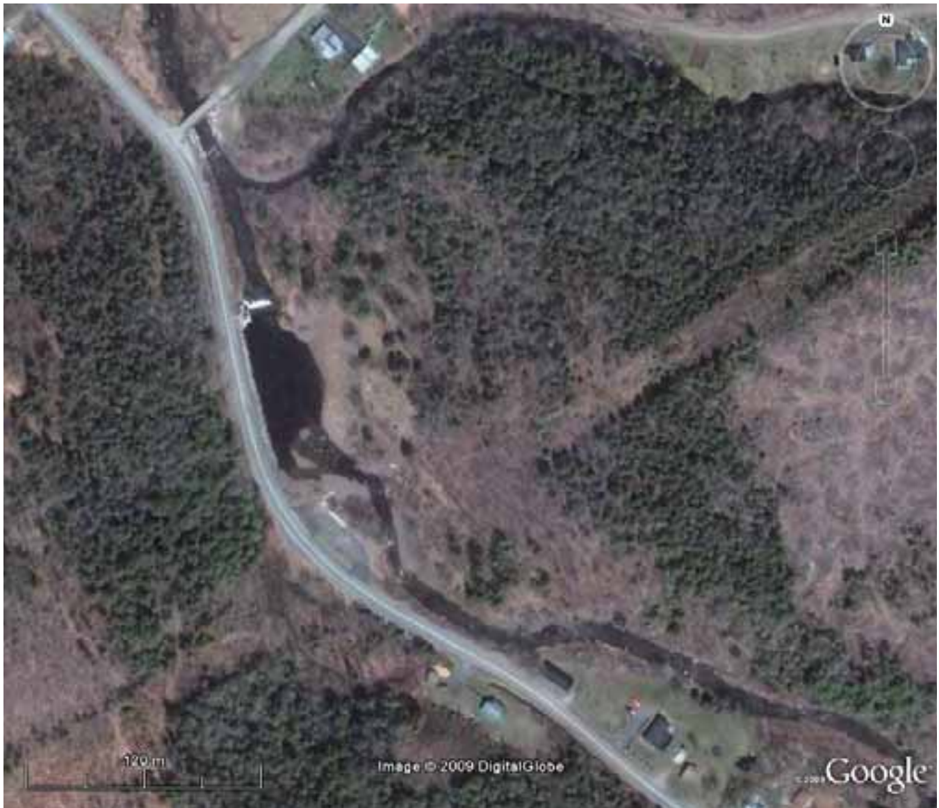
Figure 2. An aerial photo of the Clementsport dam and impoundment. Direction of water flow is from south to north. The road to the west is Clementsport Road.
