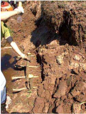
Installation of Live Sills
