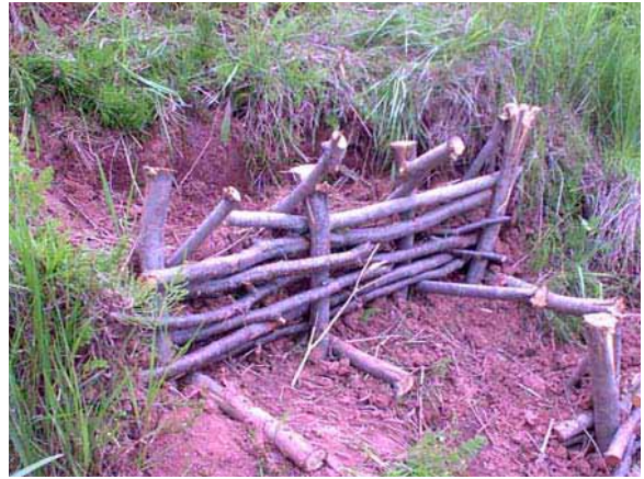
Installed Live Sills
