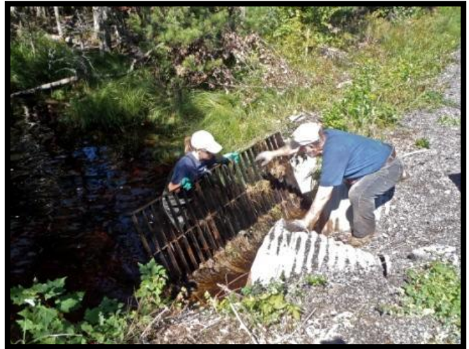
Figure 35. Removing debris blockage at inflow grate at NIC030.
