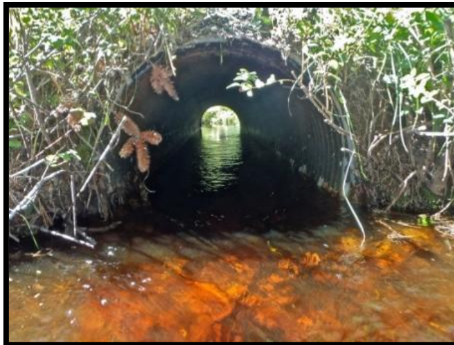
Figure 37. Third culvert at NIC030 after beaver dam removal.
