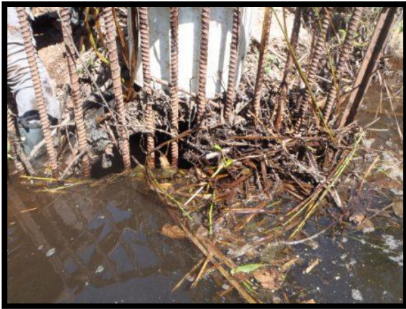
Figure 26. Debris blockage at NIC028.
