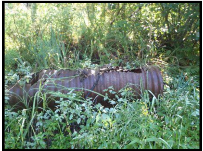
Figure 20. Evidence of a partial culvert removal at MED001.
