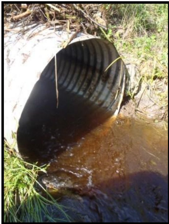
Figure 9. Water flowing through BLK013 after clearing away the beaver dam and unclogging the inflow grate.
