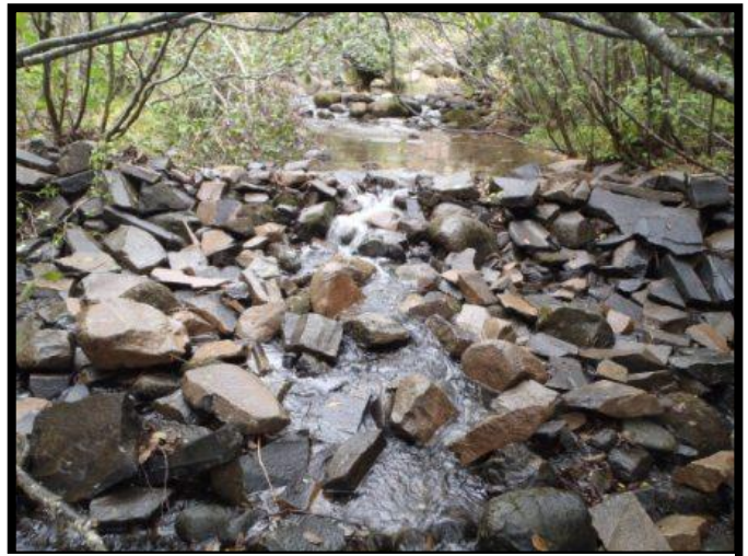
Figure 45. Weir B at TRO101 after maintenance to decrease the slope.
