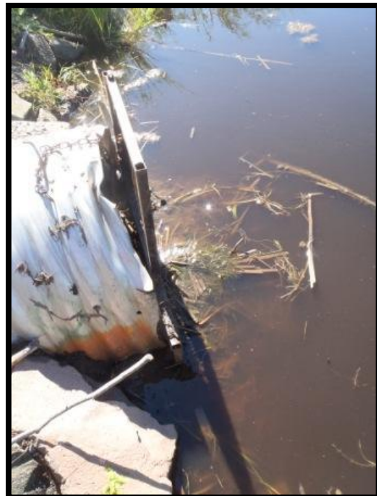
Figure 10. Vegetation build up at inflow grate at BLK031, 1 week post debris removal.
