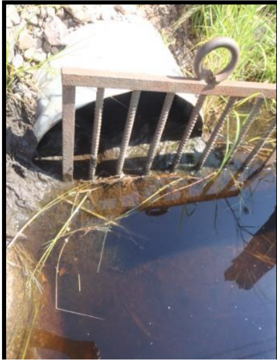
Figure 11. Vegetation and sediment build up at the inflow grate at BLK051.
