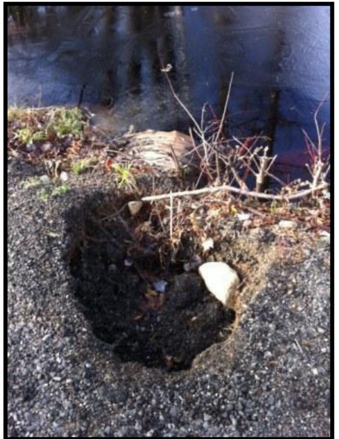
Figure 36. Shoulder of road sinking in beside third culvert at NIC030.
