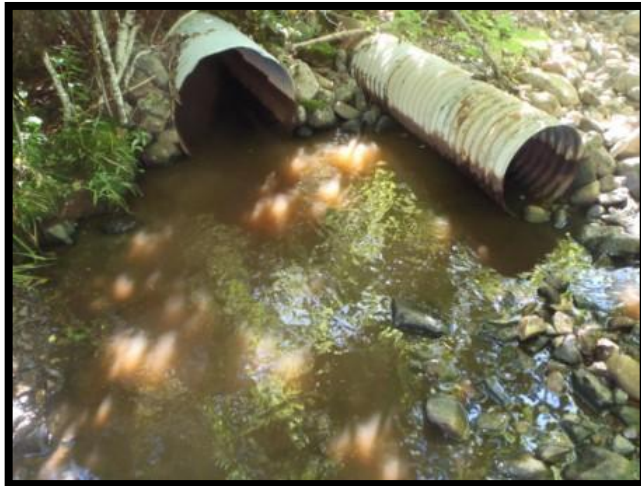
Figure 19. Two culverts at the outflow side of MED001.
