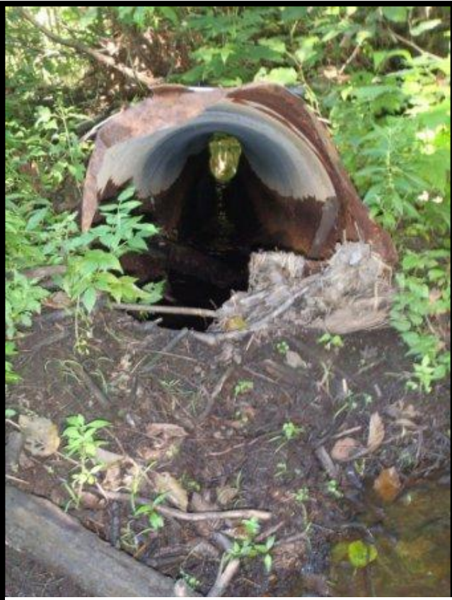
Figure 21. Debris blockage at inflow of MED001.
