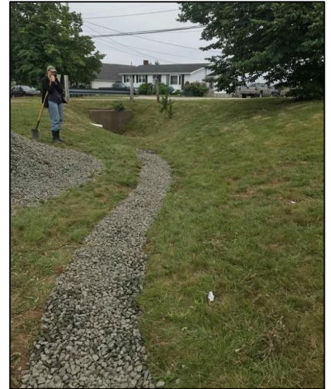
Photo description: an infiltration trench located in Digby, Nova Scotia
