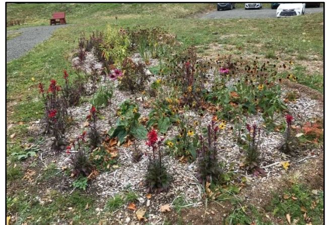
A rain garden at an LID site near the hospital located in Digby, Nova Scotia
