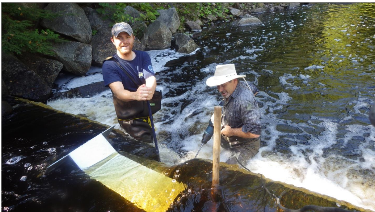
Figure 54. Preparing to install the fish chute.
