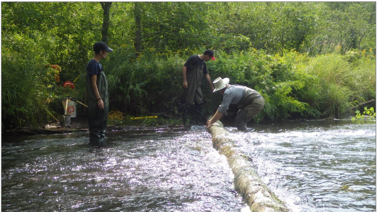
Figure 114. Fitting the log tight to the bank.
