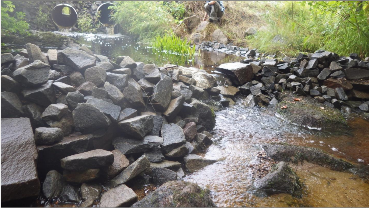
Figure 89. ALL017 Finished tailwater control weir.
