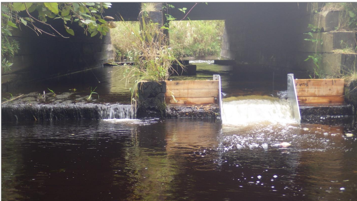
Figure 78. ROC004 Fish chute, baffles in right side, and low flow barrier at left inflow.
