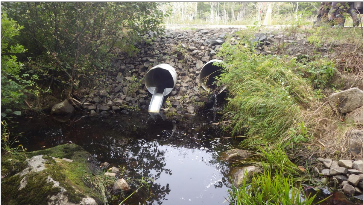
Figure 90. ALL017 after fish chute installation.
