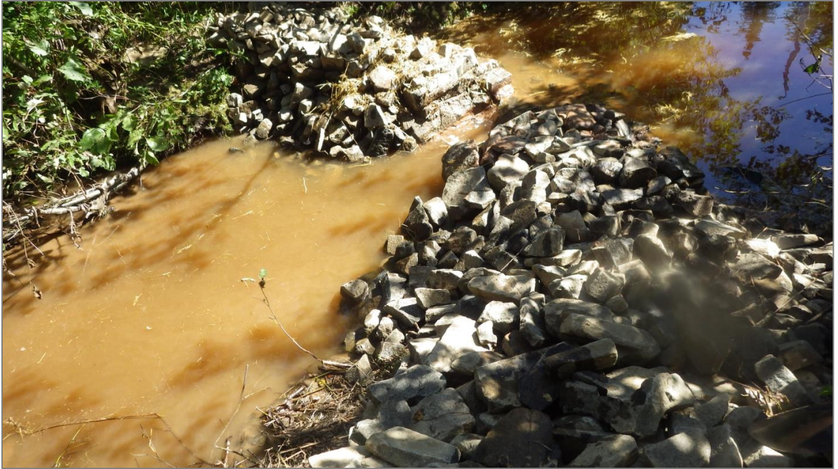
Figure 68. The completed tailwater control weir at BLK006.
