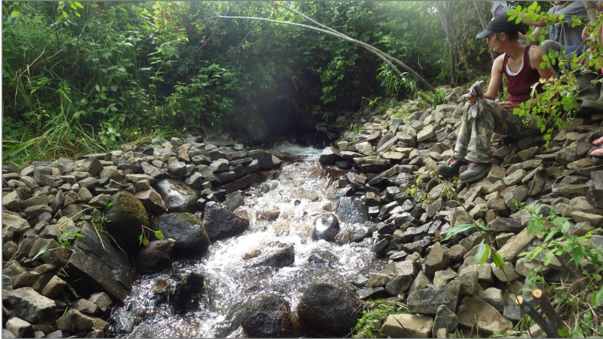
Figure 33. Completed tailwater control and bank reinforcement.
