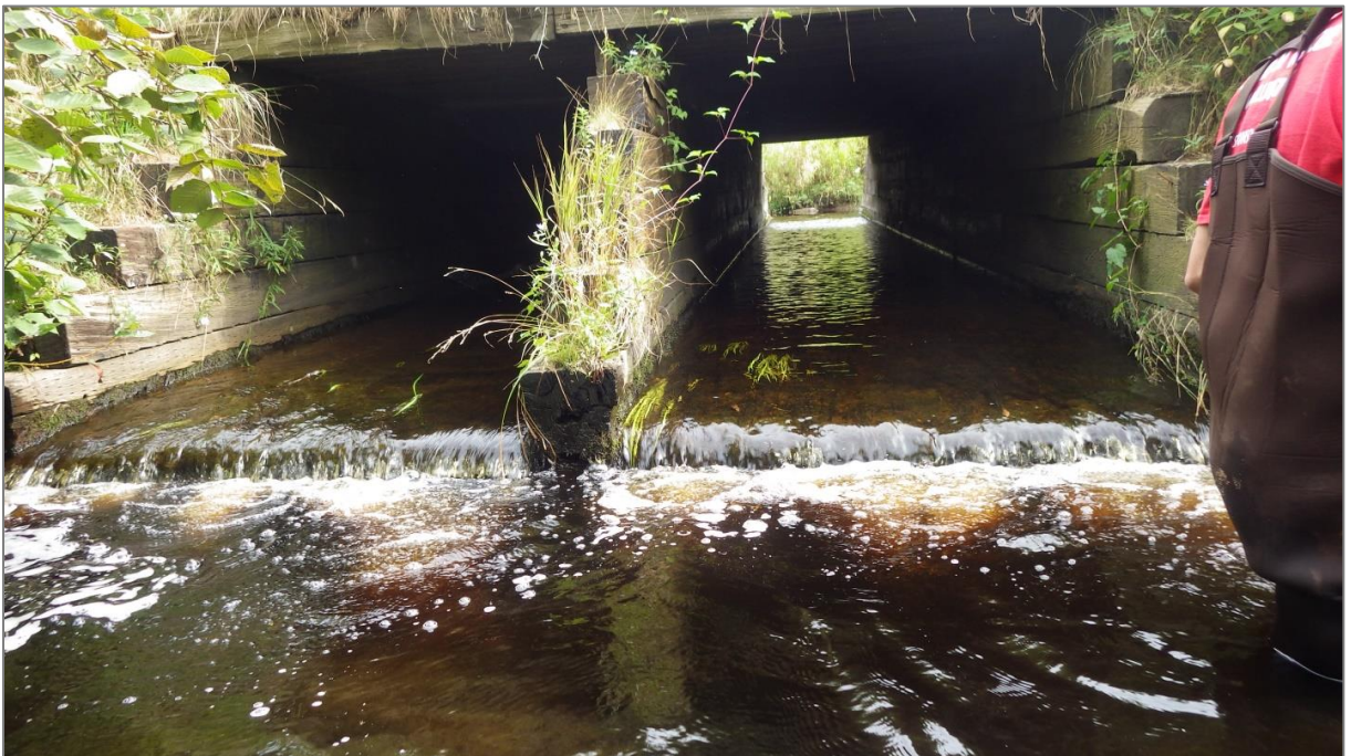
Figure 76. ROC004 Culvert after weir construction, before chute installation.
