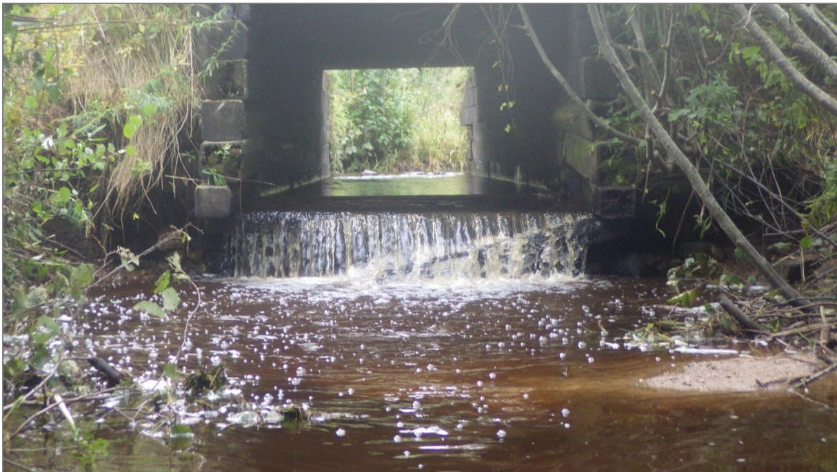
Figure 63. BLK006 Before remediation activities. Note the large outflow drop and fallen timber.
