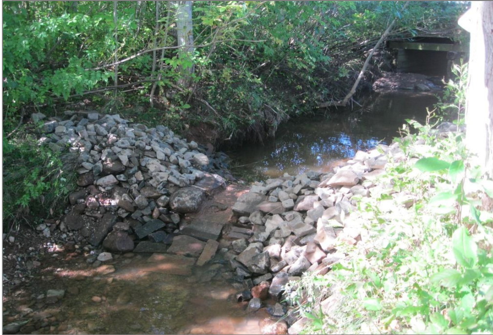
Figure 84. Finished tailwater control weir at NEB004.
