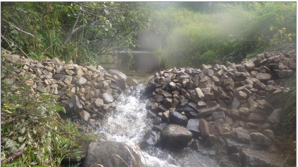
Figure 37. BAL001 First weir installed downstream of the culvert outflow.
