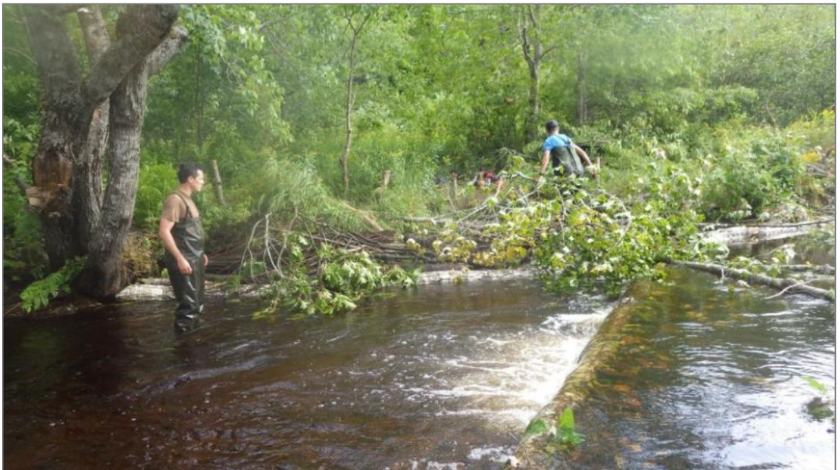
Figure 121. Reinforcing wing deflectors with trees and branches tied into the banks with stakes.
