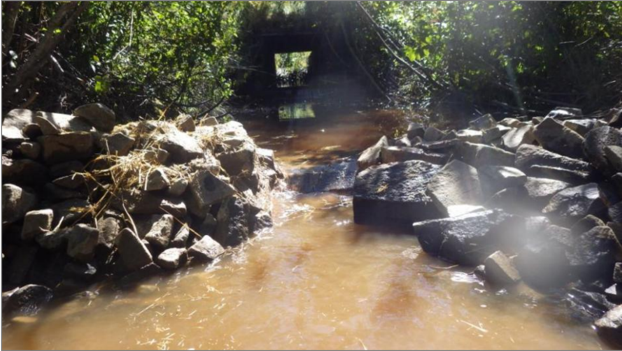
Figure 64. BLK006 After tailwater control weir construction.
