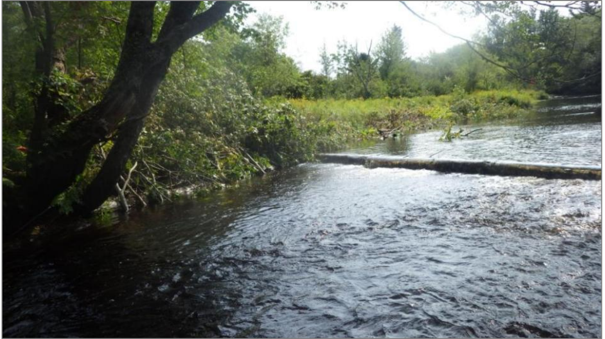
Figure 122. Completed right bank deflector.
