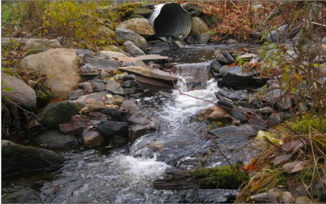
Figure 58. EAS009 After construction of tailwater control and fish chute installation.
