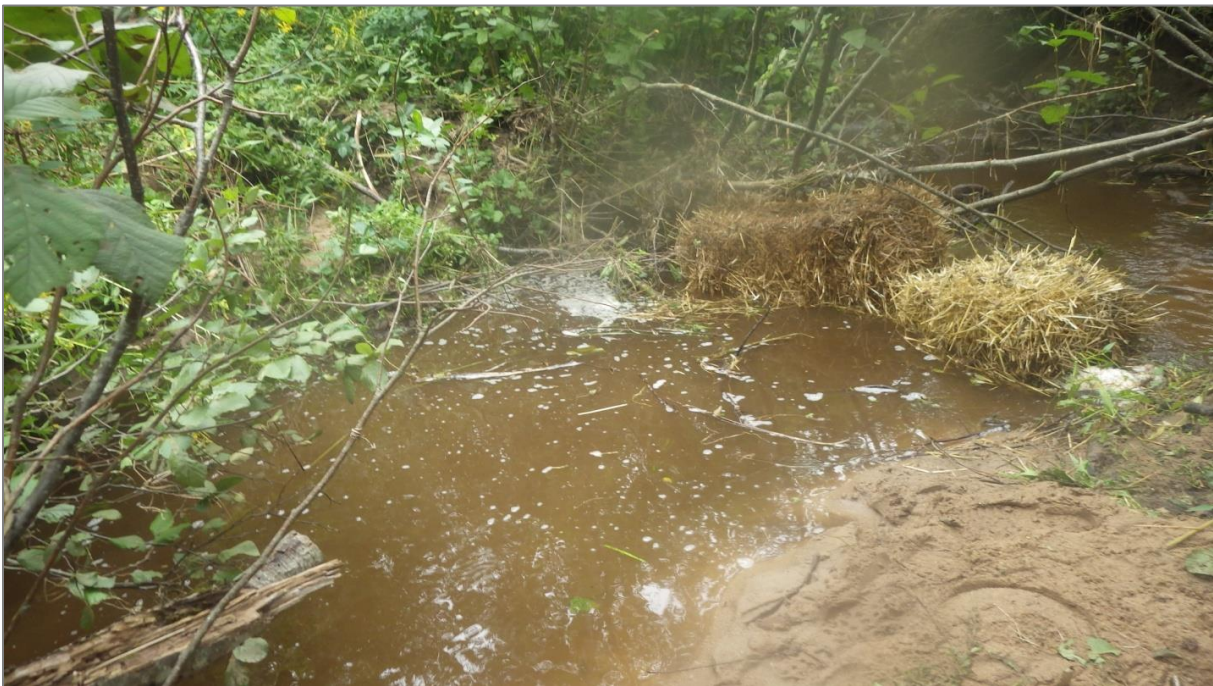
Figure 65. BLK006 Sediment trapping downstream of outflow.
