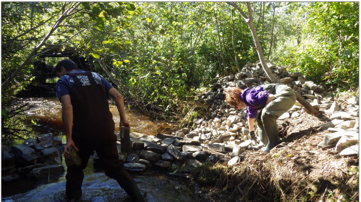
Figure 67. BLK006 Volunteer and staff building the tailwater control weir.
