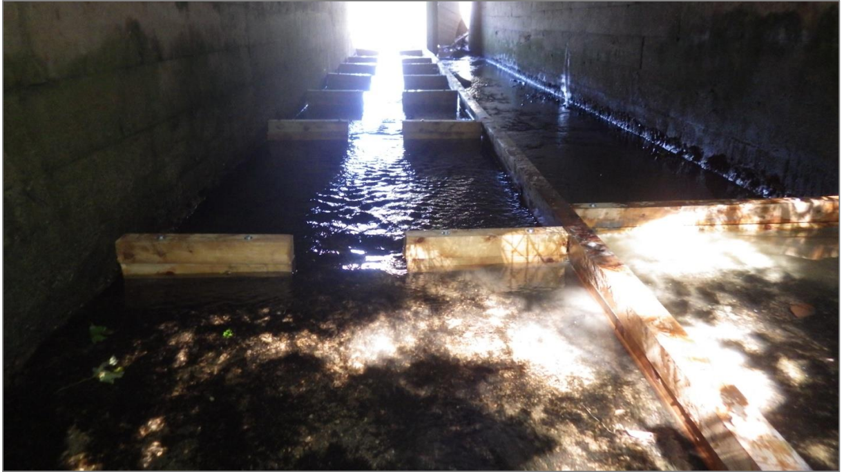
Figure 42. BAL001 Downstream view of baffles, divider, and low flow barrier.
