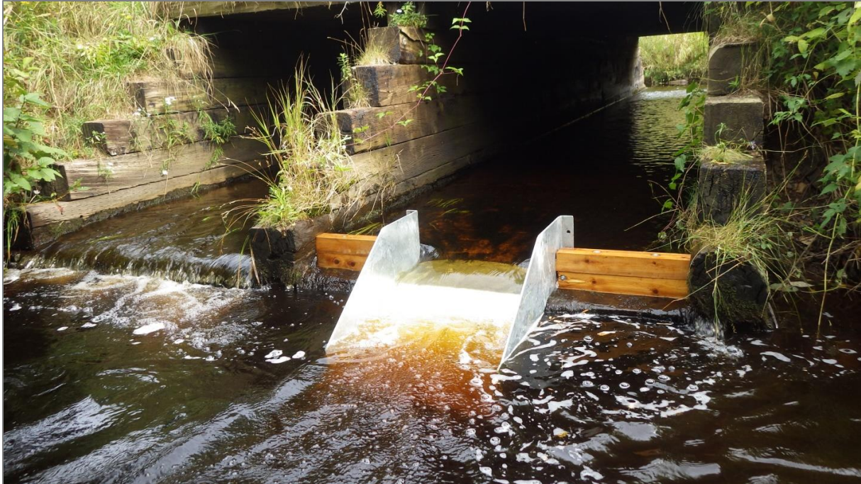
Figure 77. ROC004B After fish chute installation.
