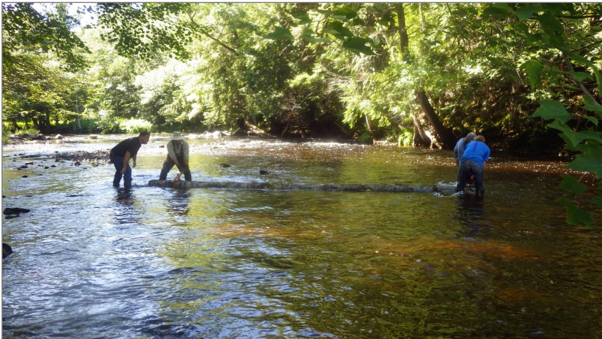
Figure 108. Log carried/floated/dragged to weir.
