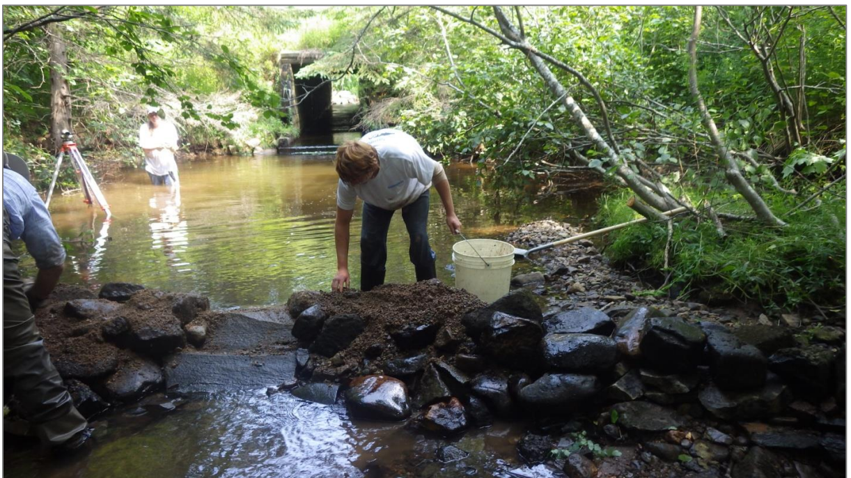
Figure 47. Construction of the tailwater control structure at MOR008.
