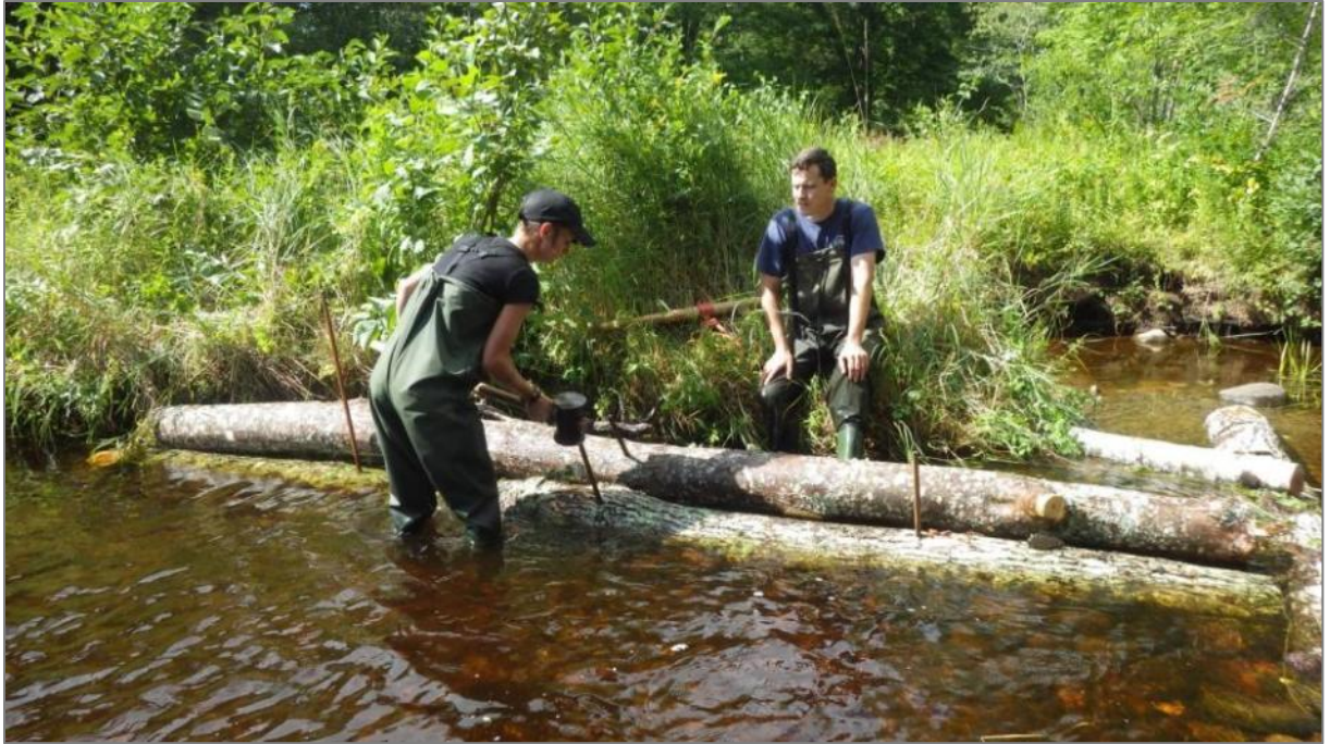
Figure 124. Securing the left bank pyramidal log structure in place.
