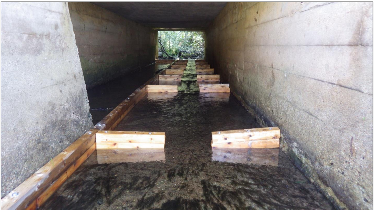
Figure 41. Baffles after installation at BAL001.
