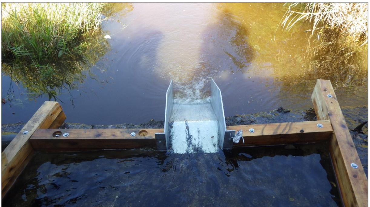
Figure 43. Fish chute after installation.
