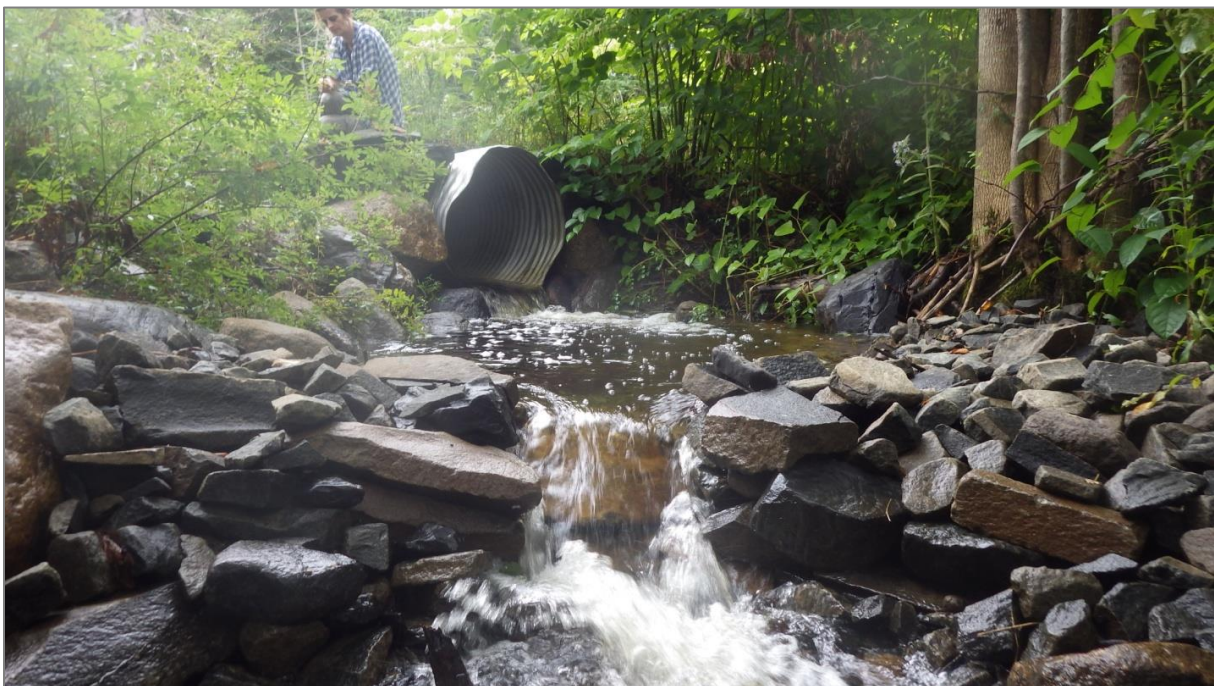
Figure 57. EAS009 After weir construction, prior to fish chute installation.
