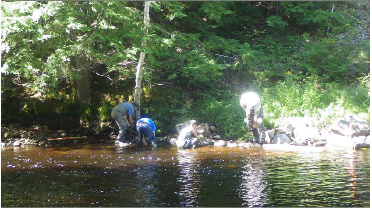
Figure 109. Crew members securing a log to the streambed as part of the installation of a wing deflector at Weir C.
