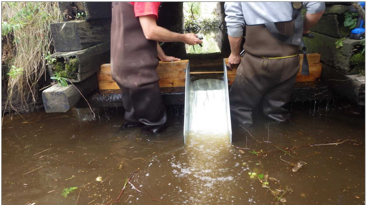
Figure 71. Fish chute at BLK006 after installation.
