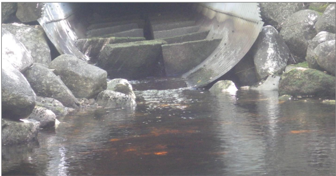
Figure 28. BUT006 Closer finished view showing derelict baffles.
