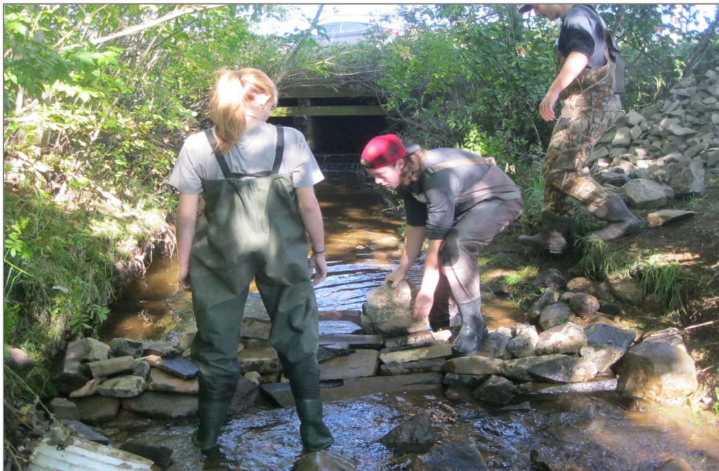
Figure 83. Volunteers hard at work constructing a rock weir at NEB004.
