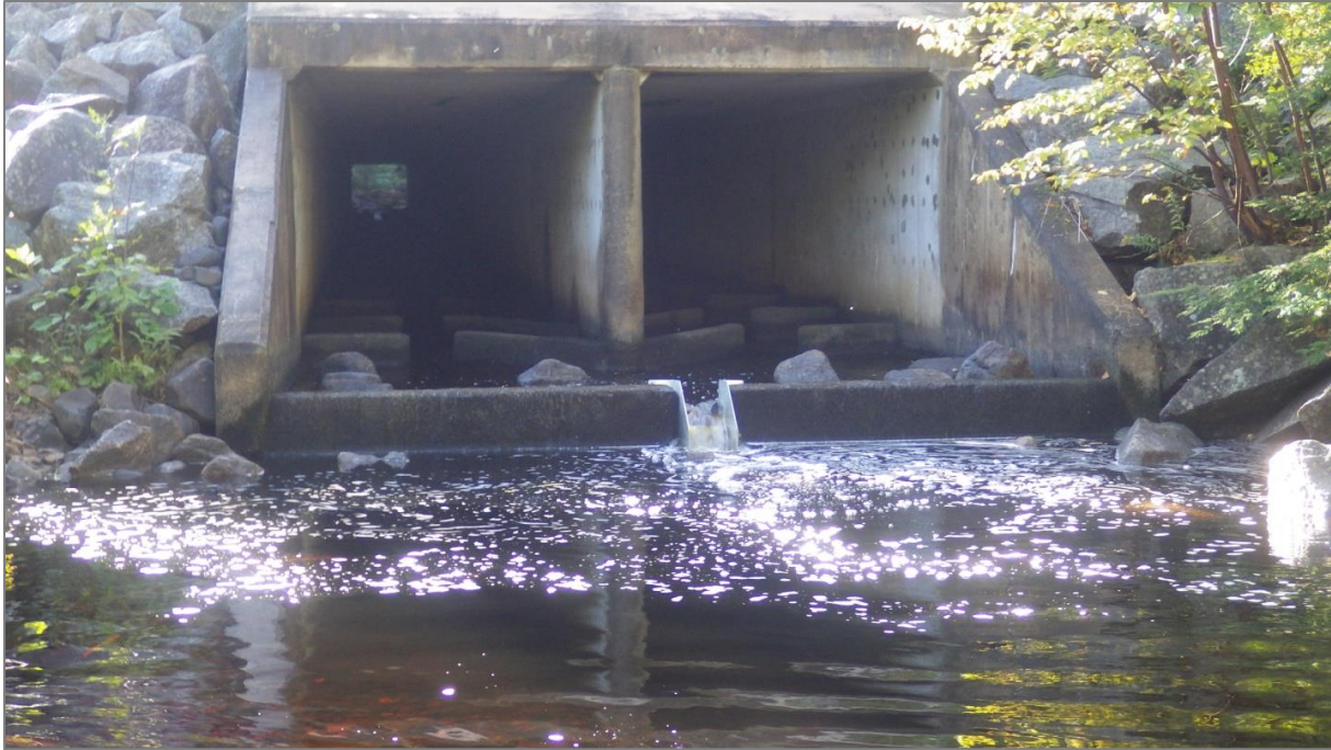
Figure 55. RHR013 after tailwater control and fish chute installation were complete.
