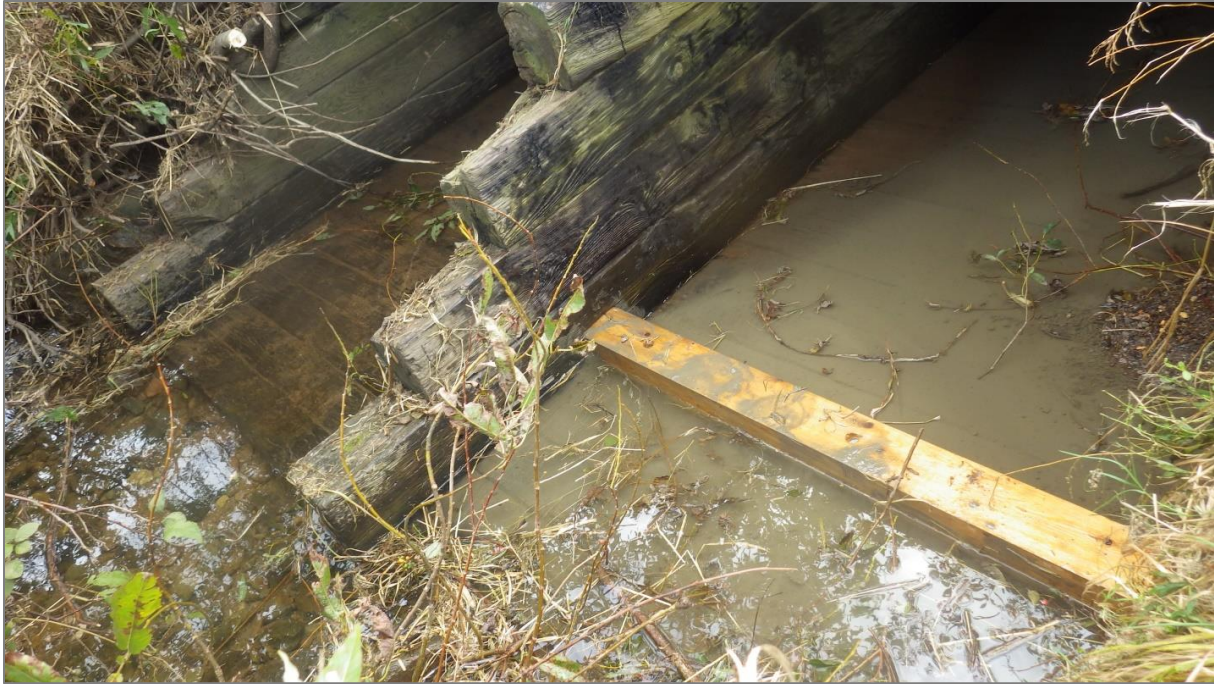
Figure 86. NEB004 after installation of a low flow barrier at the inflow.
