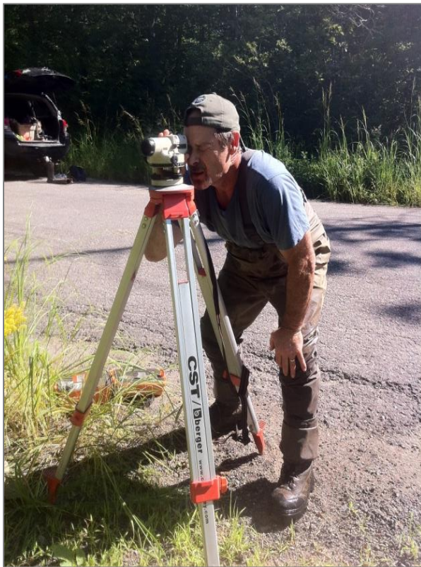
Figure 59. Checking height of culvert to set notch stone.
