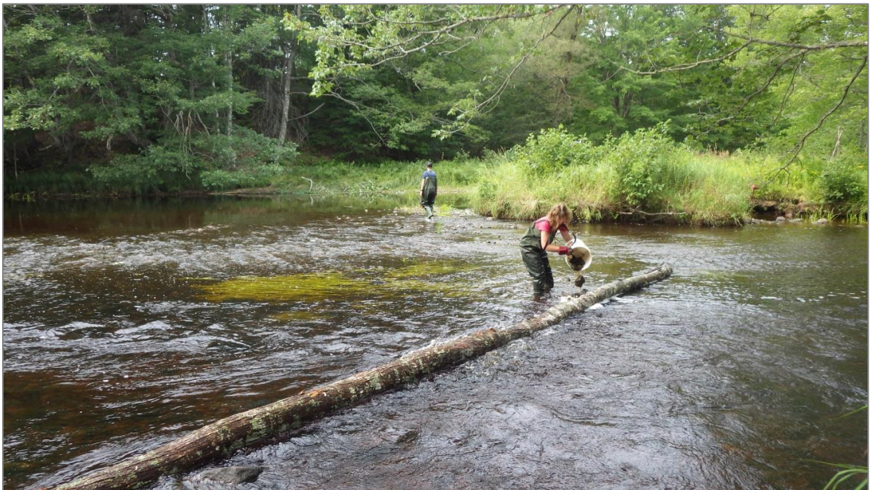
Figure 116. Placing rocks on the upstream side of the digger log.
