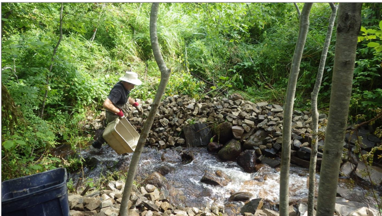
Figure 32. Reinforcing the banks at site NIC002.
