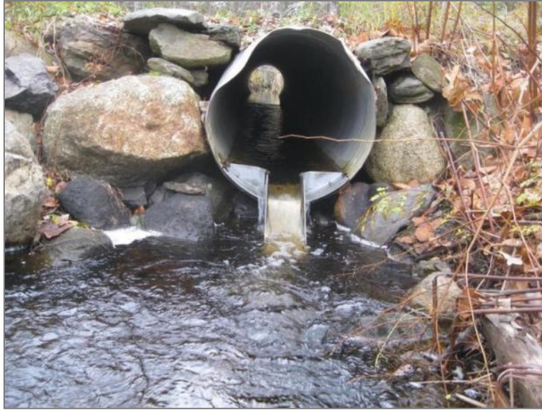
Figure 61. View of functioning fish chute after installation at EAS009.
