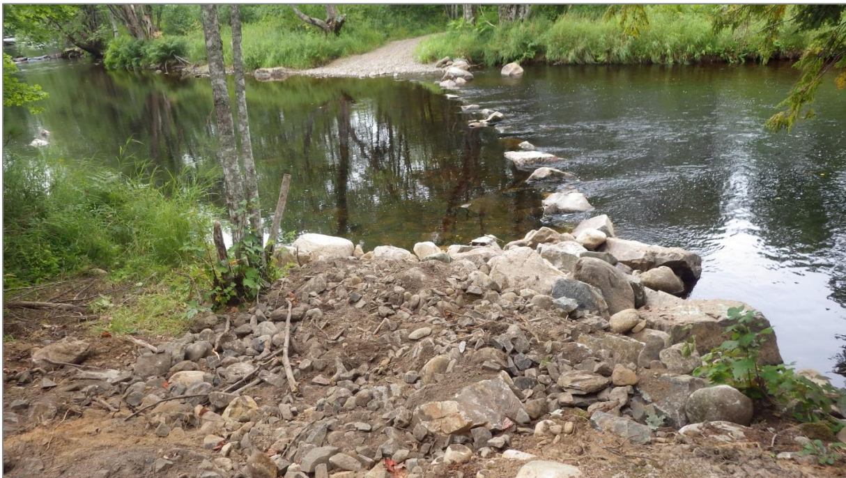
Figure 105. Weir "G" after the addition of the right wing deflector.
