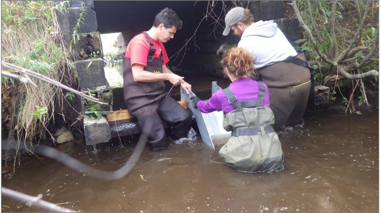
Figure 70. Installing the fish chute at BLK006 with help from Adopt-A-stream staff.
