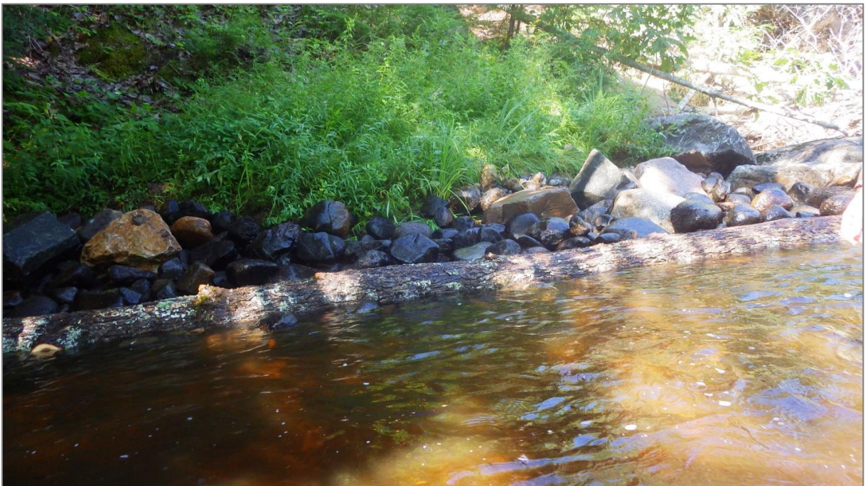
Figure 110. Finished wing deflector.
