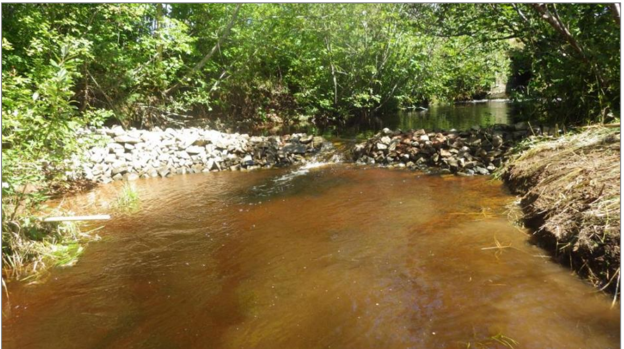
Figure 74. ROC004 Completed tailwater control weir.
