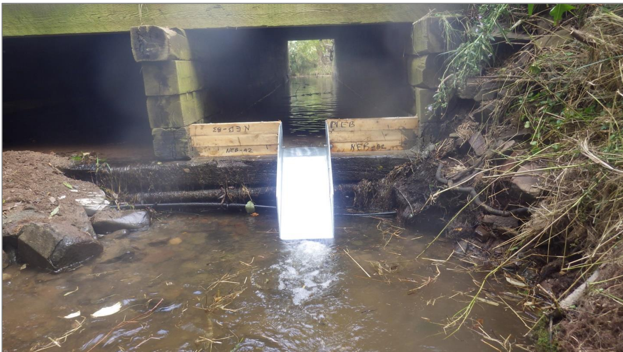
Figure 85. NEB004 after fish chute installation.
