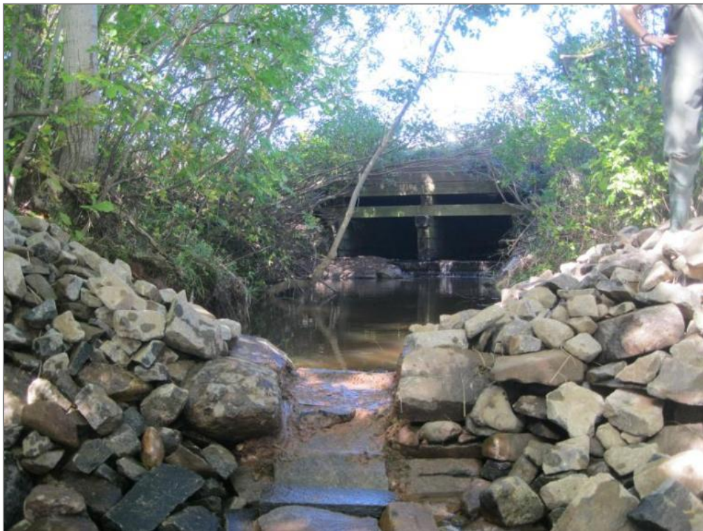
Figure 81. NEB004 After tailwater control weir installation.
