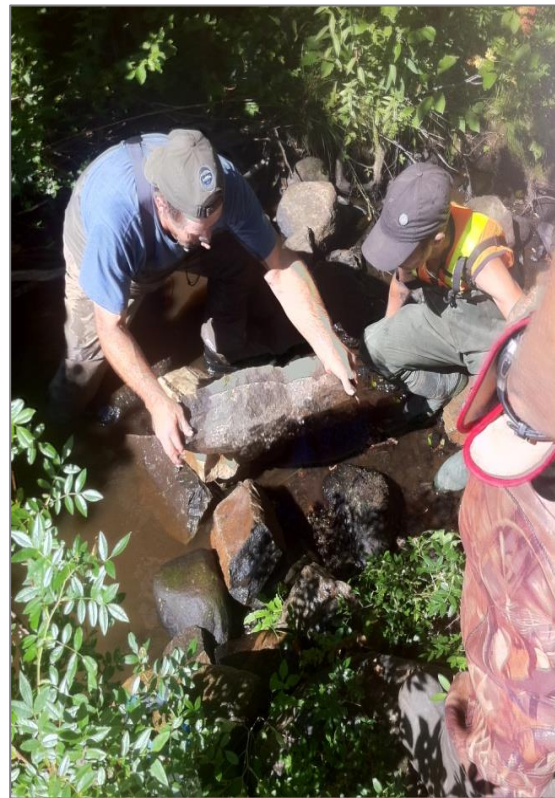
Figure 60. Construction of the tailwater control weir at EAS009.
