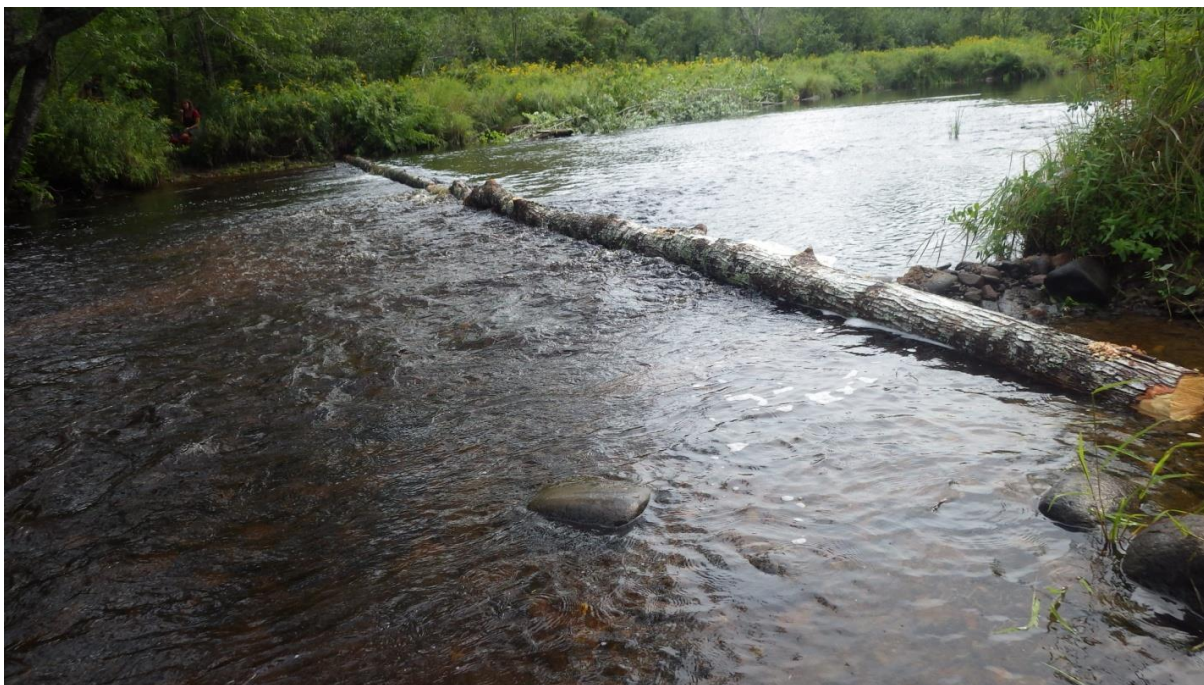
Figure 117. Finished double digger log structure, prior to installation of wing deflectors.
