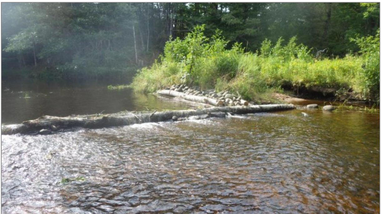
Figure 125. Left bank deflector finished.
