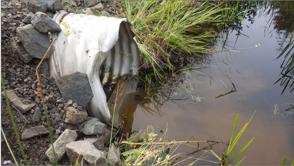
Figure 91. ALL017 Installation of low flow barrier at culvert inflow (culvert without the fish chute).
