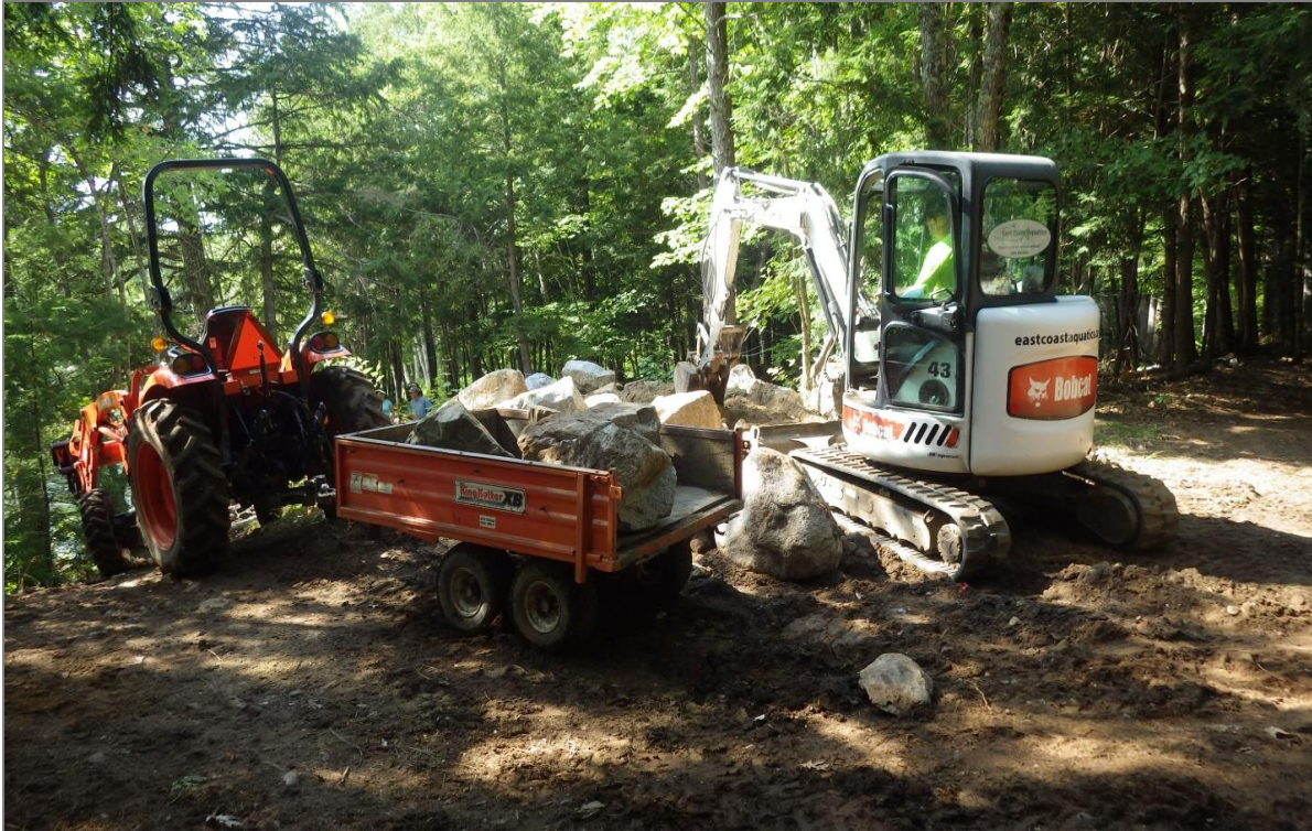
Figure 92. Excavator and tractor used to move weir rocks to weir sites.
