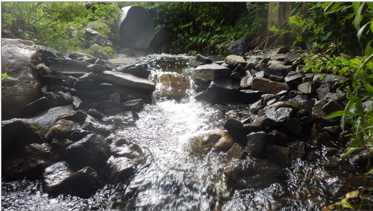
Figure 62. A small pool was created below the weir at EAS009 to improve fish access.
