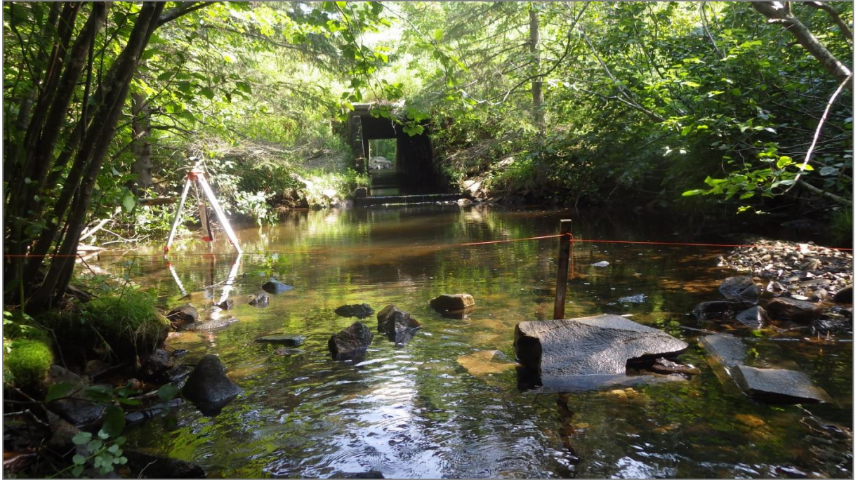
Figure 46. Measuring out the placement of the downstream rock weir.
