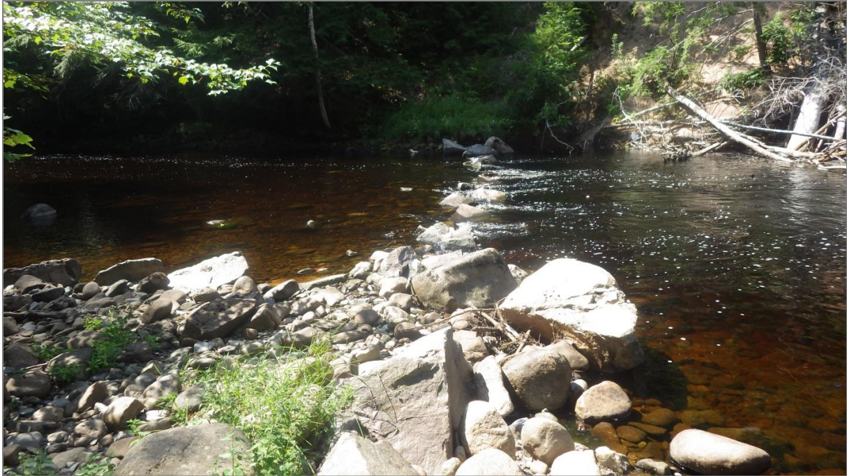
Figure 98. Weir "C" Before wing deflector adjustments.
