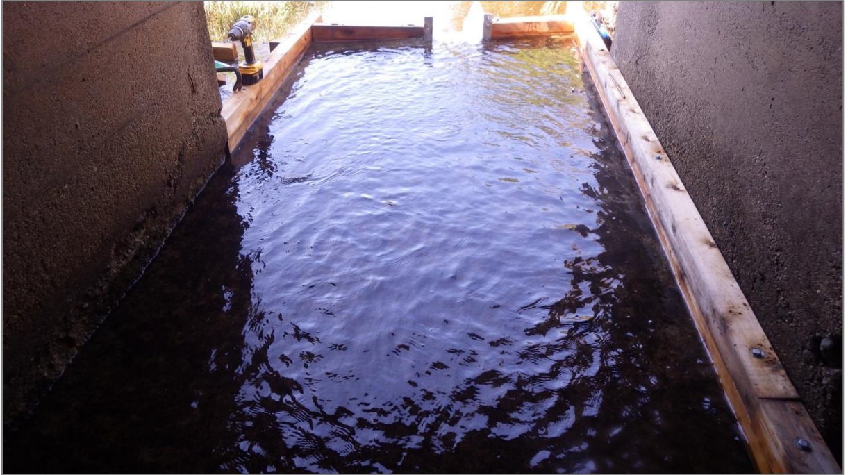
Figure 40. BAL001 Newly created divider, ready for baffles and fish chute installation.
