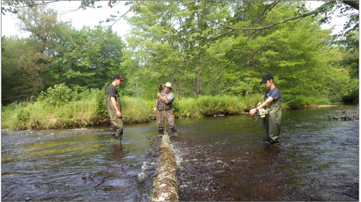
Figure 115. Logs were secured to the streambed using re-bar.
