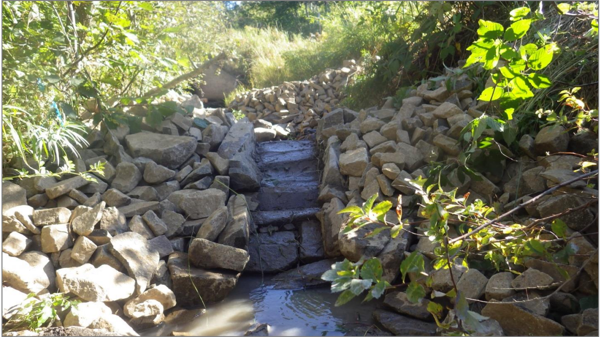
Figure 38. BAL001 Second weir, downstream of culvert outflow and first weir, after completion.
