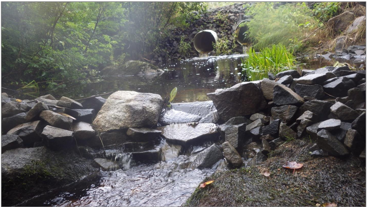
Figure 88. ALL017 After tailwater control weir construction.
