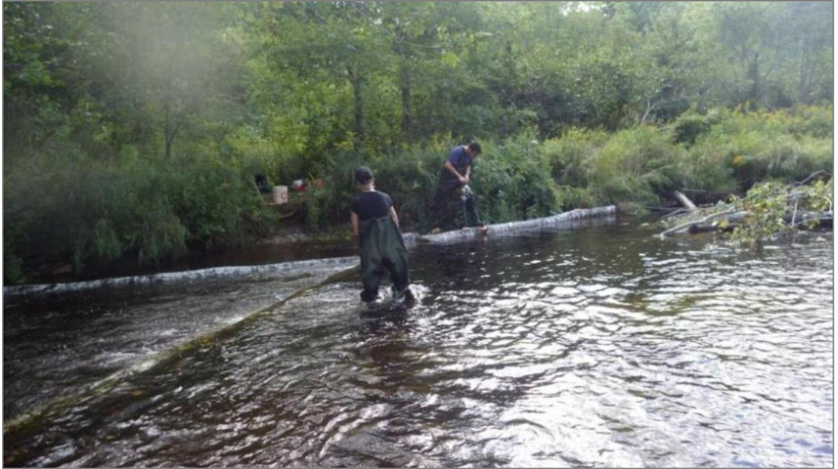
Figure 120. Upstream triple log portion of the left wing deflector during the installation process.
