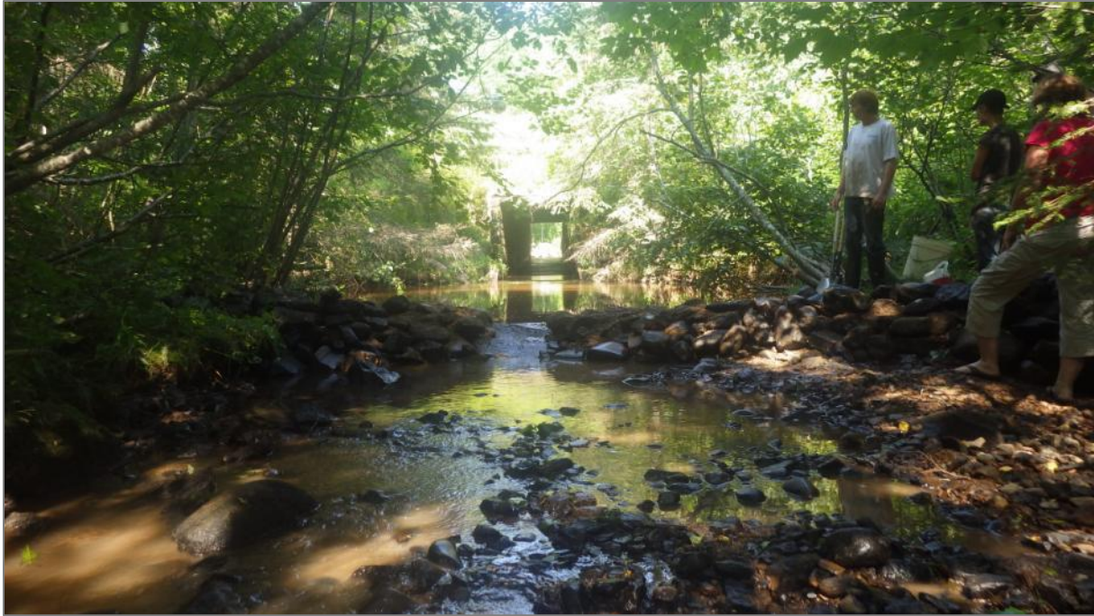
Figure 48. Completed tailwater control structure.
