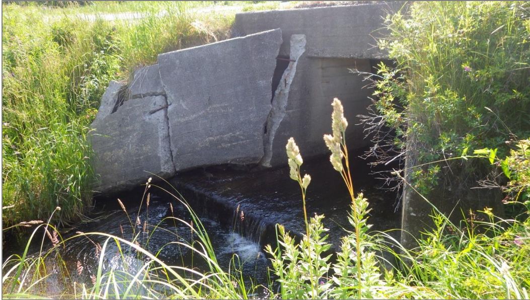
Figure 34. BAL001 Broken concrete divider that requires removal.
