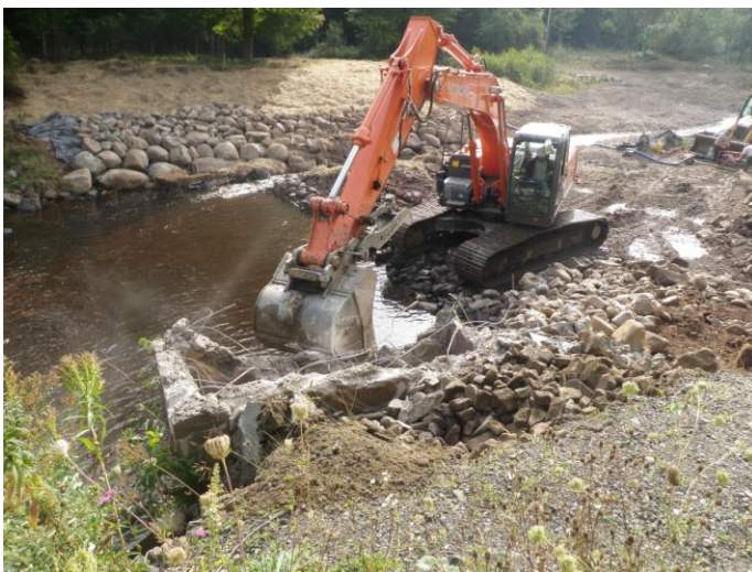
Figure 6 | Demolition of concrete abutment.
