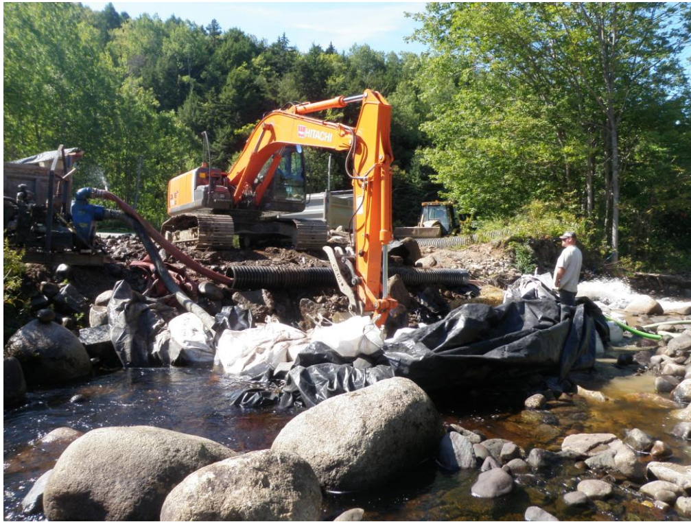
Figure 8 | Stabilizing an eroding bank upstream of the impoundment area.
