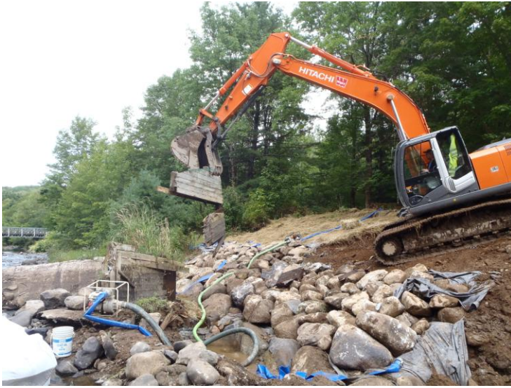
Figure 4 | Removal of fish ladder.
