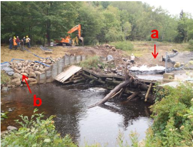
Figure 2 | Silt and erosion control measures established at the dam removal site. Silt fences are denoted by a) and b) shows some bank protection measures put in place.
