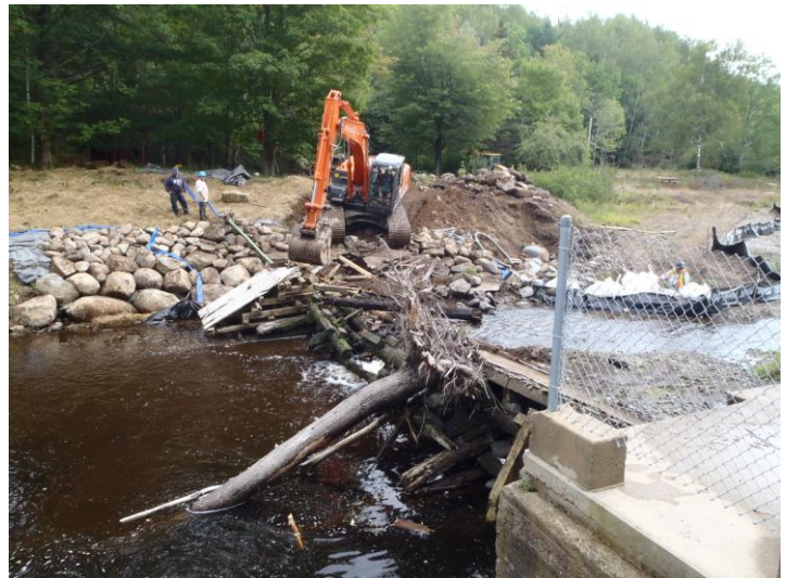
Figure 5 | Removal of wooden crib structure.
