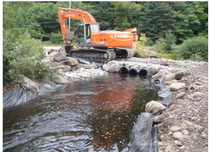
Figure 3 | Diversion channel during dam removal.
