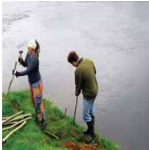
Figure 2- Willow staking May 2009 at the Town of Middleton site.
