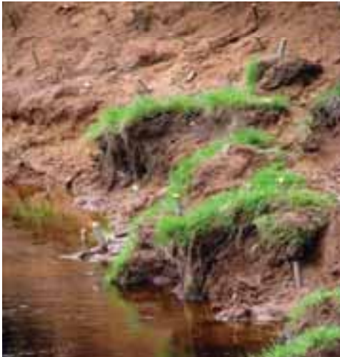
Figure 1- Willow stakes providing bank stabilization at the Town of Middleton site.
