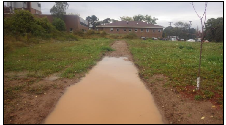
Post rain event at stormwater demonstration site in Digby, Nova Scotia
