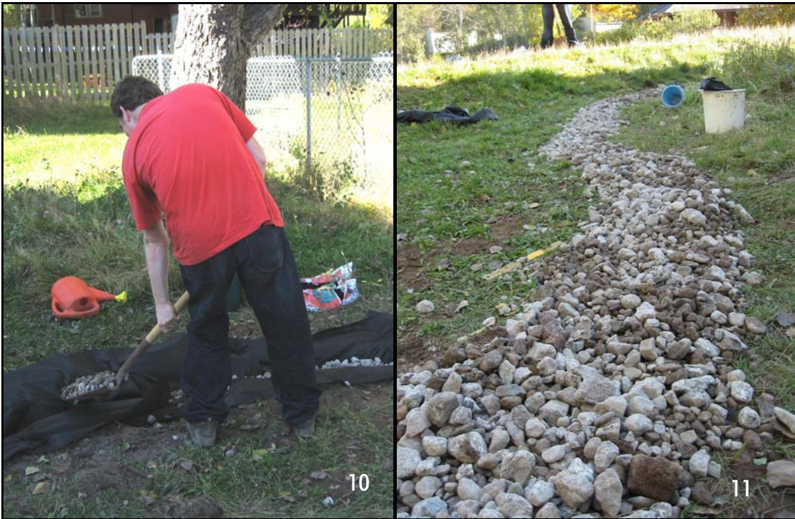
Figure B10. Laying the rock in the dry creek bed.
