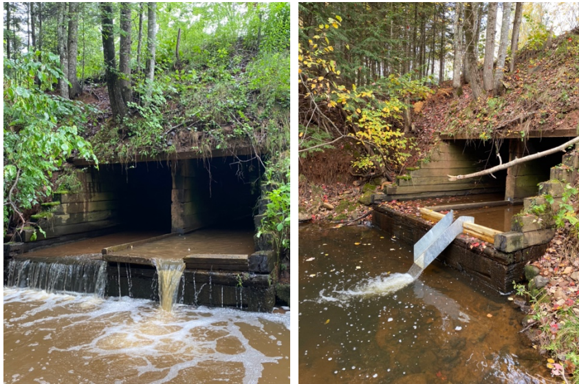
Figure 32. WAT004 before (left) and after (right) the fish chute installation.
