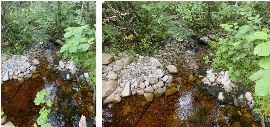
Figure 23. Rock weir built at EAL001.
