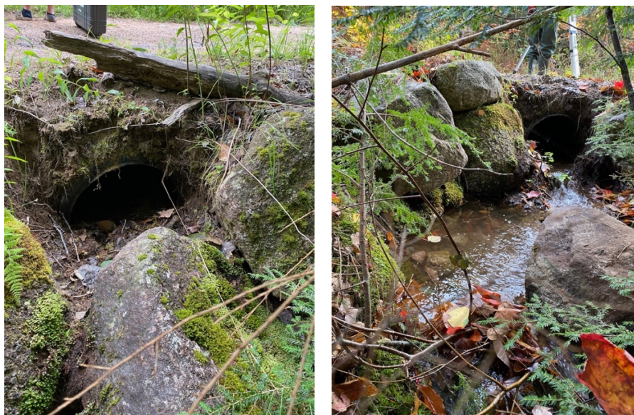
Figure 7. Before (left) and after (right) of the culvert outflow debris removal.
