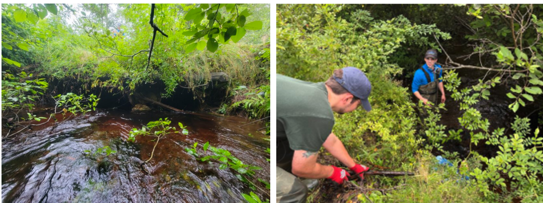
Figure 37. SHB006 before (left) and during (right) the debris removal.
