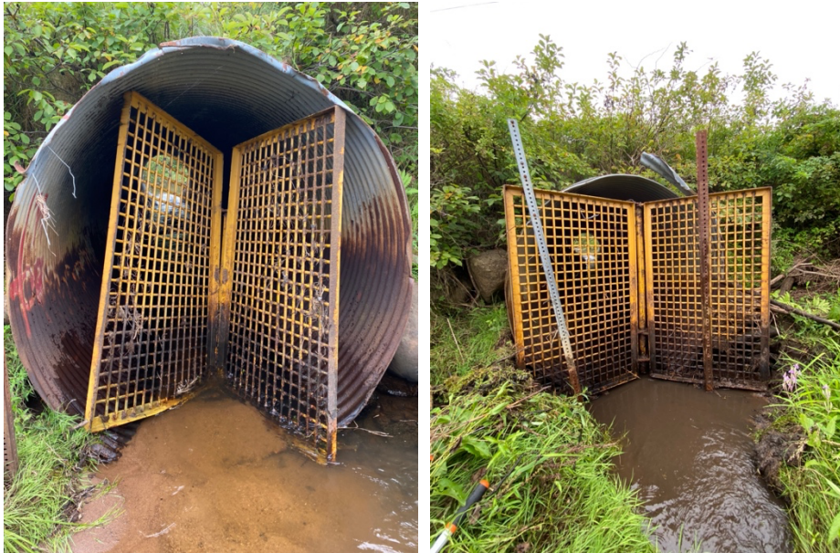
Figure 35. TRO010 inflow after the debris removal.
