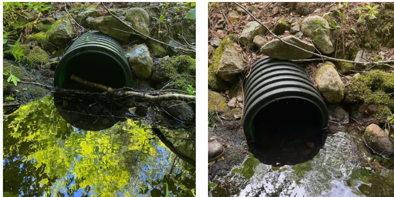
Figure 14. FAL013 before (left) and after (right) debris removal.
