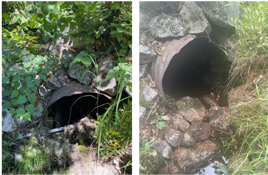
Figure 16. CLO001 before (left) and after (right) debris removal.
