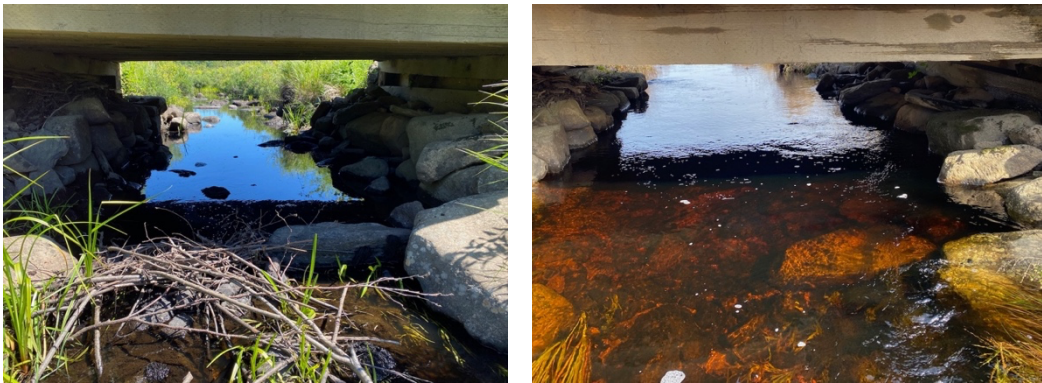
Figure 10. NEW001 before (left) and after (right) debris removal.
