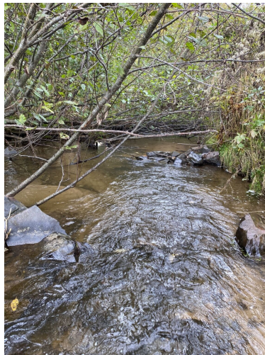
Figure 25. The rock weir at RFB001 no longer intact.
