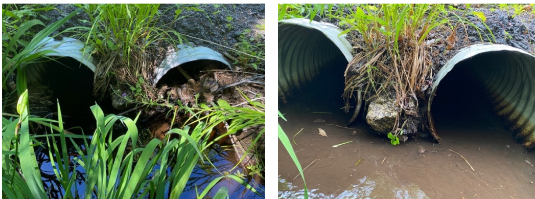
Figure 15. RHR064 before (left) and after (right) debris removal.
