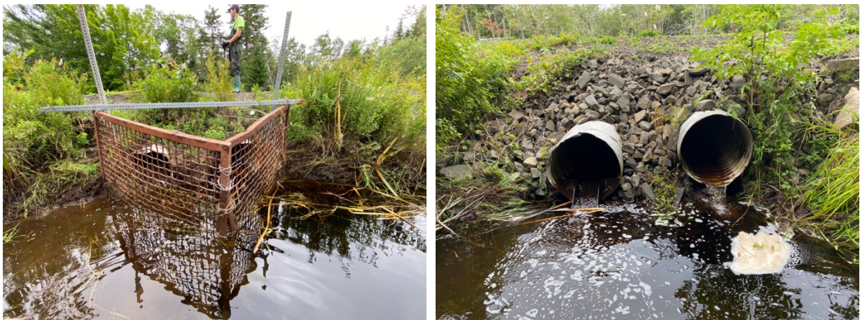
Figure 30. ALL017 inflow (left) and outflow (right) after the debris removal.
