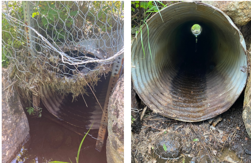
Figure 18. RHR061 before (left) and after (right) debris removal.
