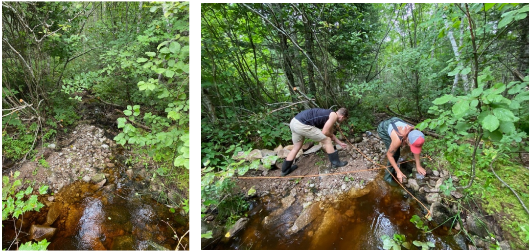
Figure 22. EAL001 before rock weir construction.
