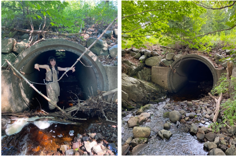
Figure 31. PET002 before (left) and after (right) debris removal.
