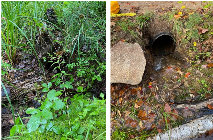
Figure 6. Before (left) and after (right) the culvert inflow debris removal.
