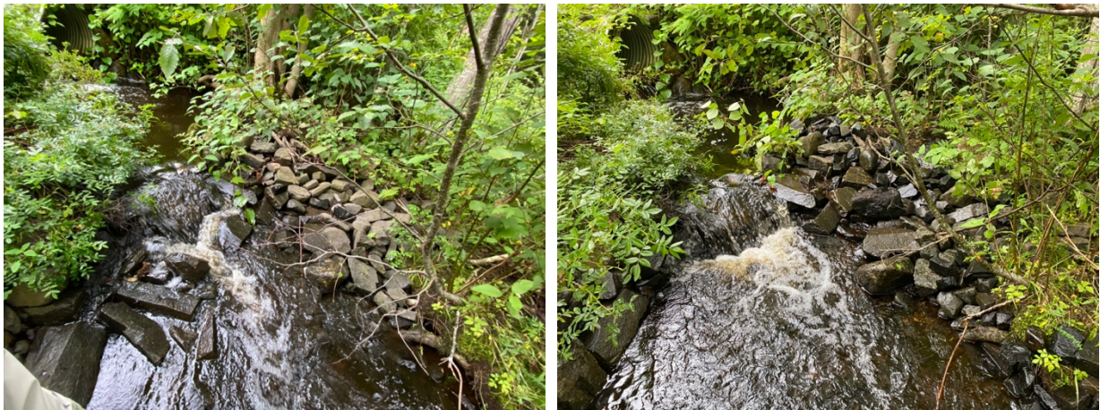
Figure 28. Before (left) and after (right) the tailwater control structure maintenance.
