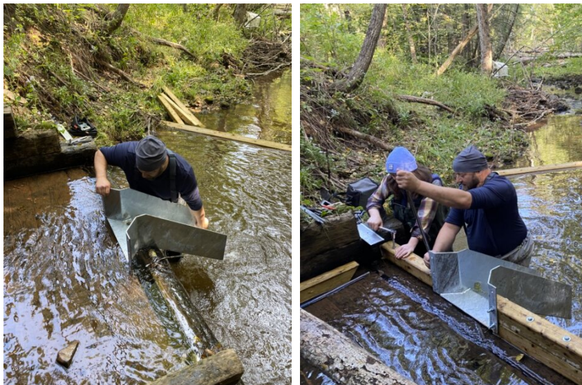
Figure 33. CARP staff, Levi Cliche and Shauna Forrestall installing the fish chute.
