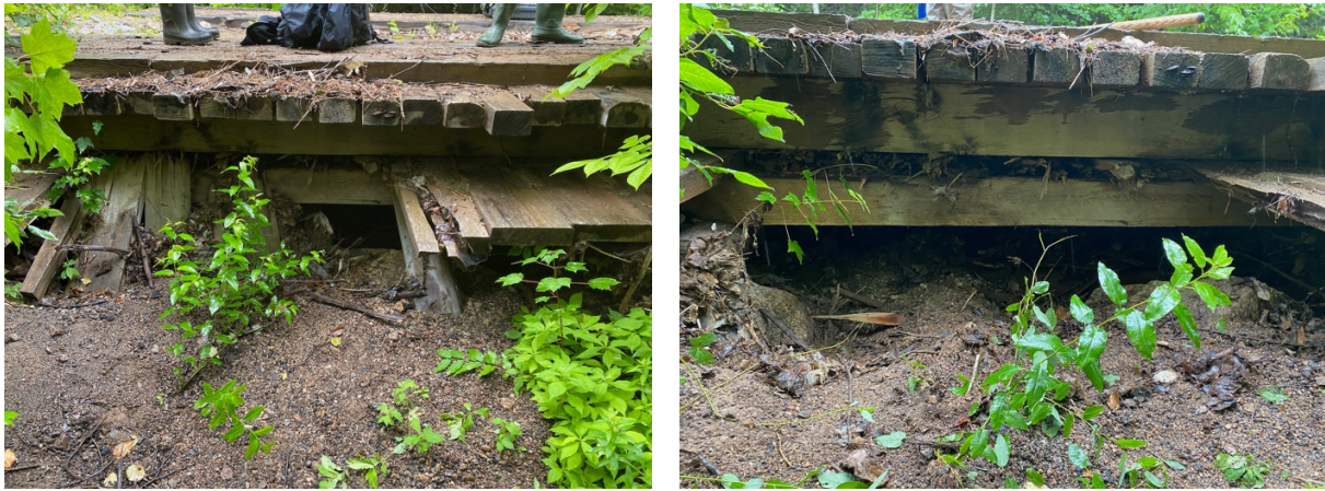
Figure 8. BIG002 before (left) and after (right) debris removal.
