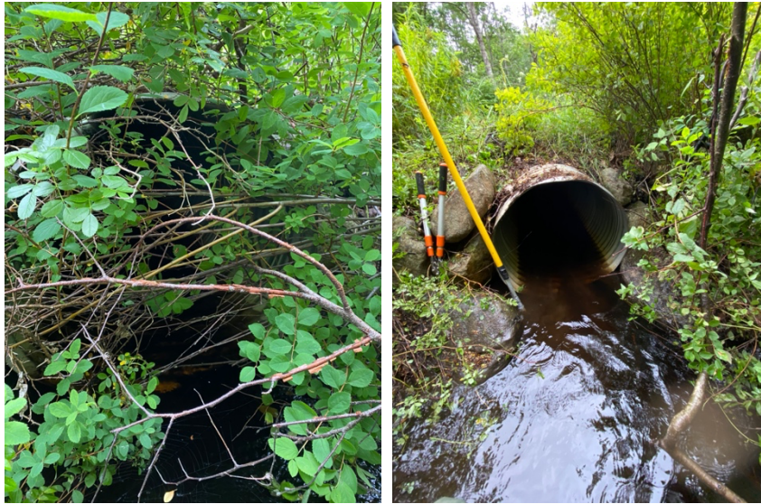
Figure 27. EAS009 before (left) and after (right) the culvert inflow debris removal.
