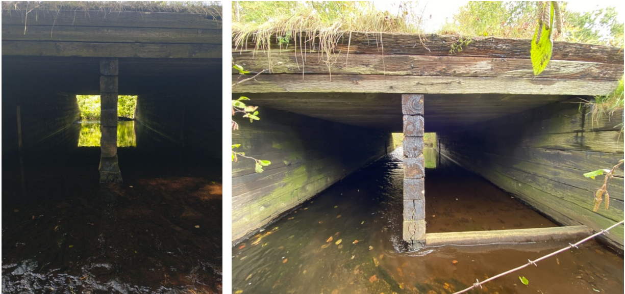
Figure 26. SHB005 before (left) and after (right) the low-flow barrier installation.
