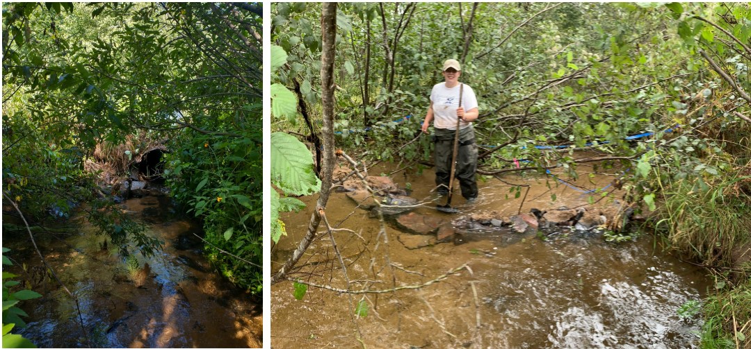
Figure 24. RFB001 before (left) and during (right) rock weir installation.
