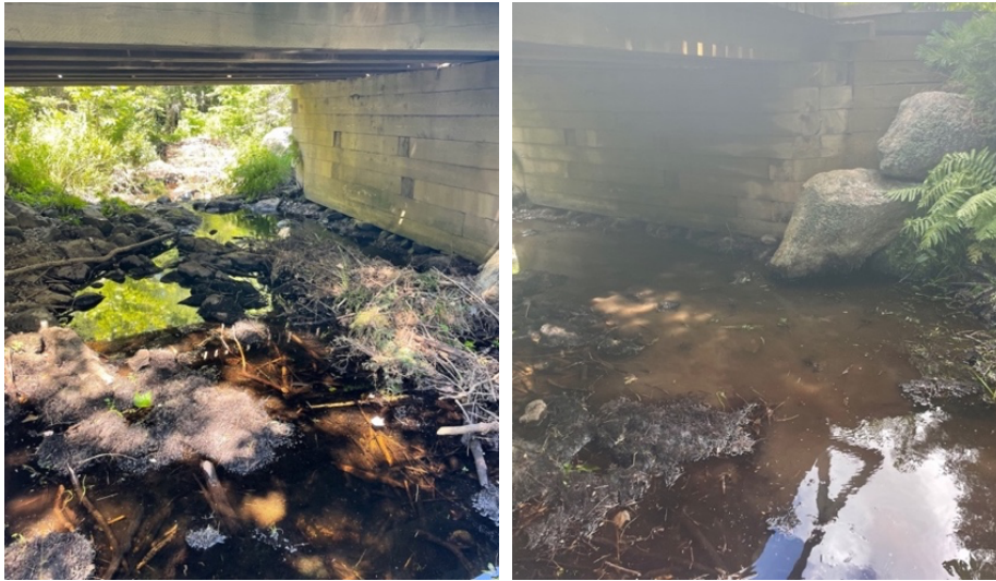
Figure 12. MAR001 before (left) and after (right) debris removal.
