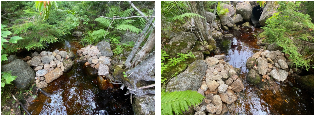
Figure 21. Rock weir built on Joudrey Brook.
