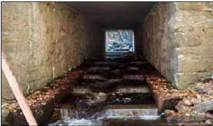
Figure 3: A concrete baffle system to reduce flow velocities and/or increase water depth in culvert (Source: CTDEP Inland Fisheries, 2008)
