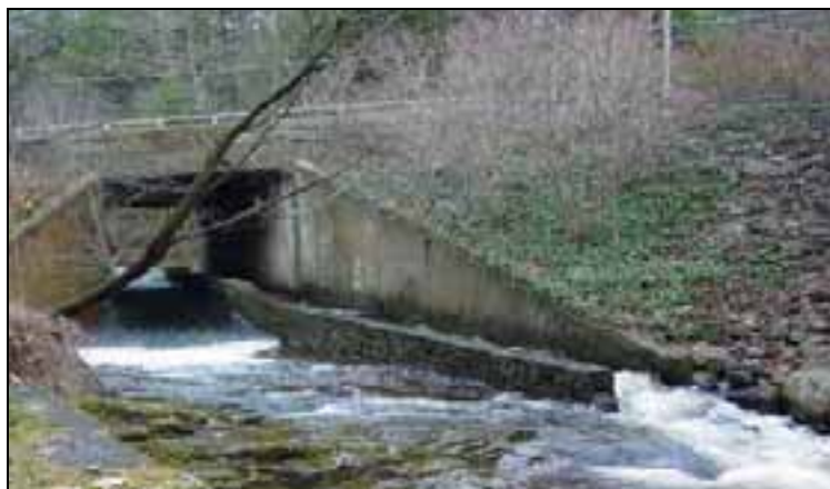
Figure 5: A fishway installed within a culvert to facilitate fish passage (Source: CTDEP Inland Fisheries, 2008)
