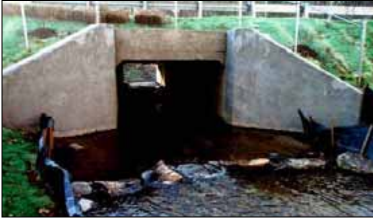
Figure 2: A tailwater control weir backing up water to eliminate outfall drop and/or increase water depth in culvert (Source: CTDEP Inland Fisheries, 2008)
