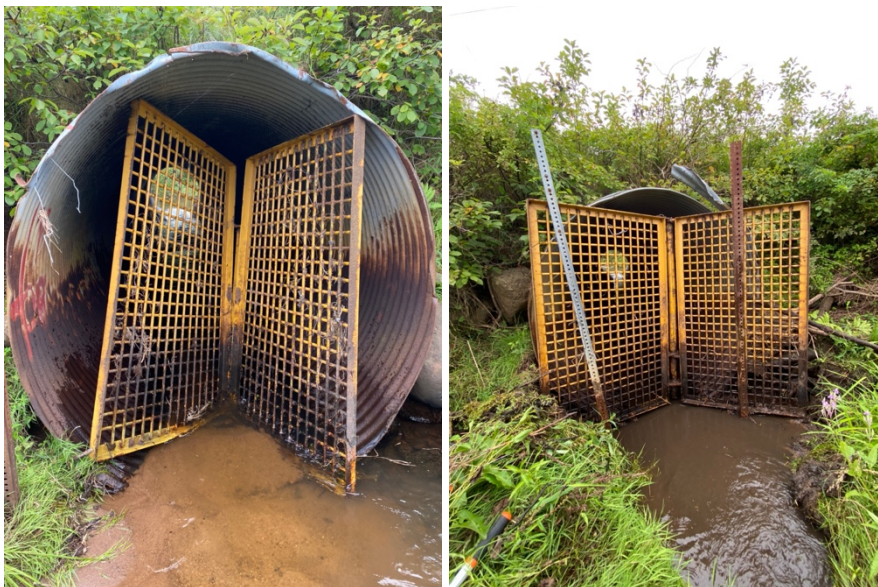
Figure 14. TRO010 inflow after the debris removal.
