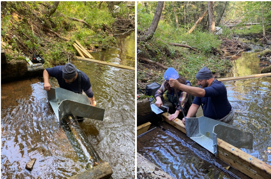
Figure 12. CARP staff Levi Cliche and Shauna Forrestall installing the fish chute.
