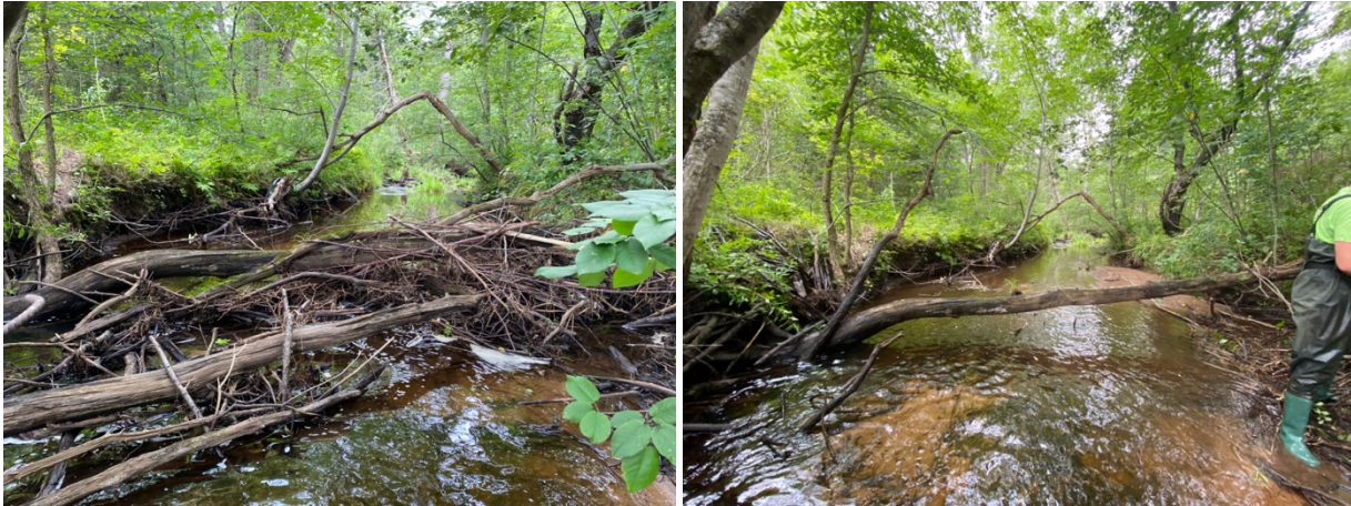
Figure 15. Downstream of BLK004 before (left) and after (right) debris removal.
