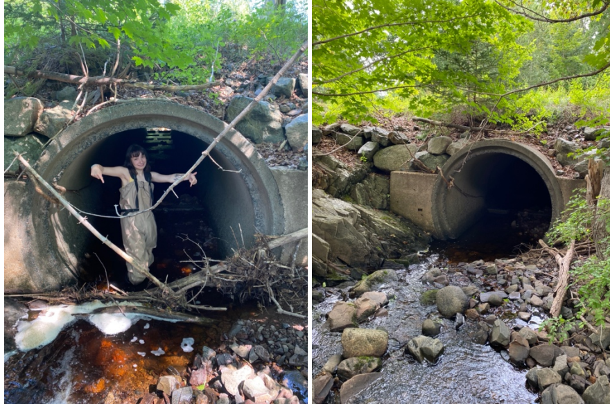
Figure 10. PET002 before (left) and after (right) debris removal.
