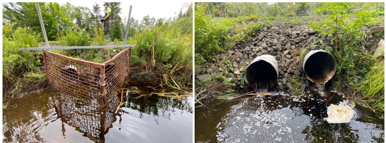
Figure 9. ALL017 inflow (left) and outflow (right) after the debris removal.
