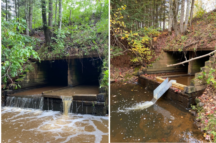
Figure 11. WAT004 before (left) and after (right) the fish chute installation.
