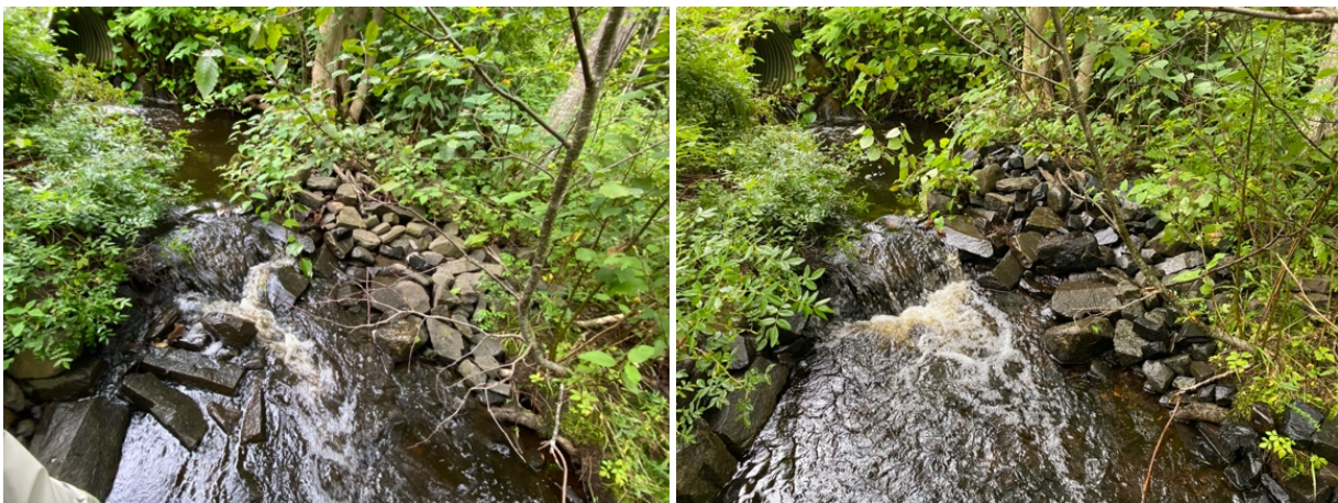
Figure 7. Before (left) and after (right) the tailwater control structure maintenance.
