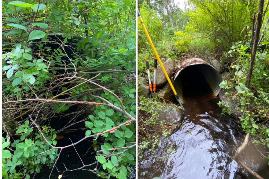
Figure 6. EAS009 before (left) and after (right) the culvert inflow debris removal.
