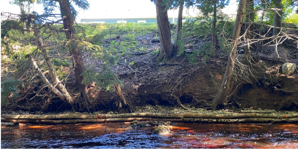
Figure 8. Log crib installed to protect an eroding bank along the Fales River.
