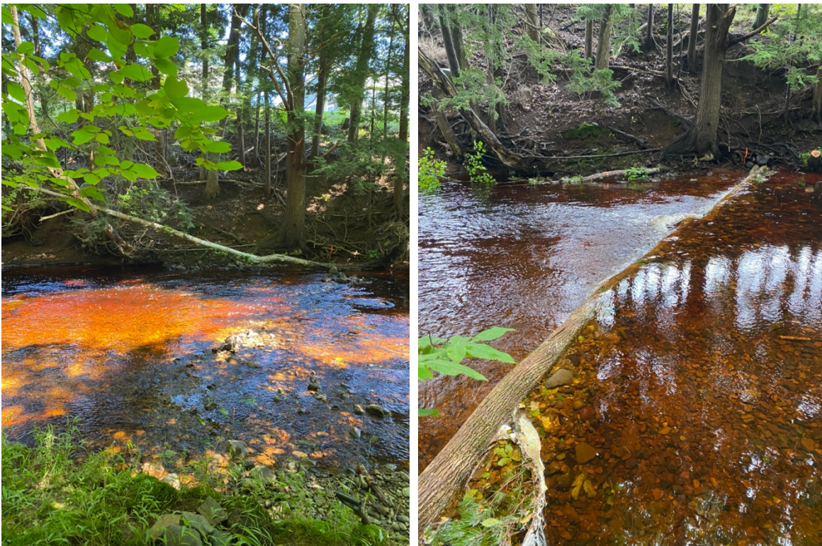
Figure 9. Before (left) and after (right) digger log installation on the Fales River.
