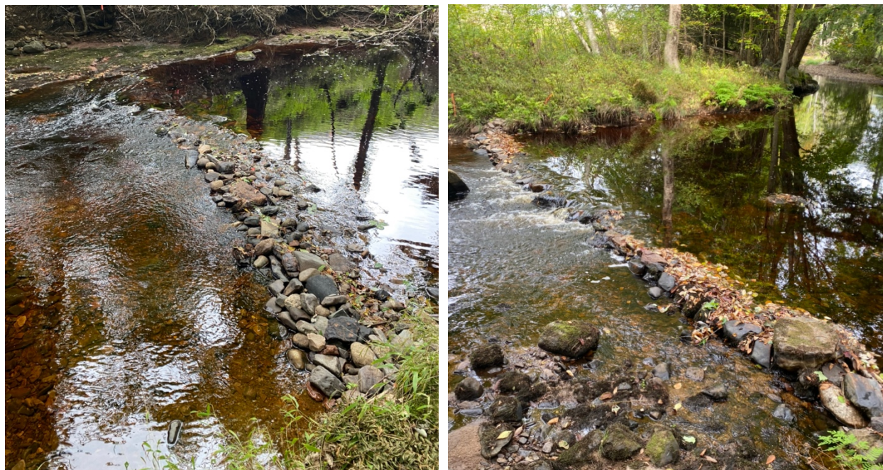
Figure 10. Two rock sills installed along the Fales River.
